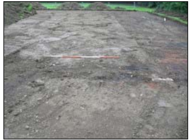
Plate 4: Looking south across area of new netball court
