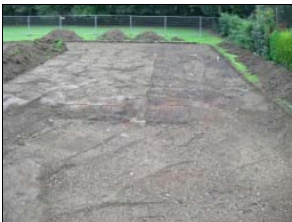
Plate 5: View south across hard court cleared of topsoil
