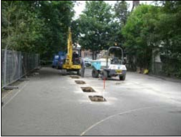
Plate 1: View NW along western side of foundations
