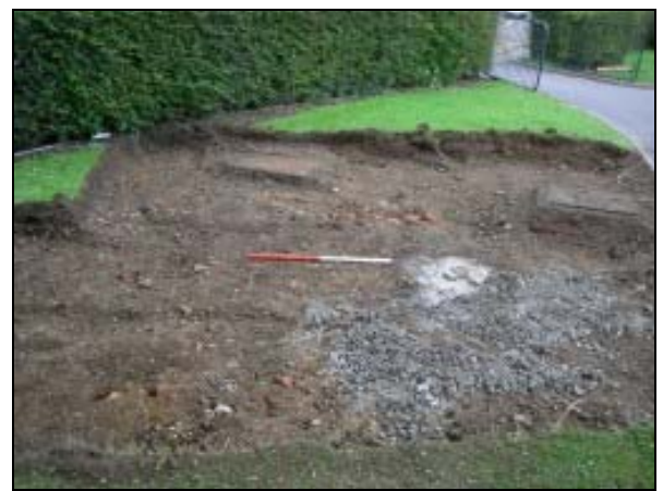
Plate 6: View north of new parking bay to the west of school
