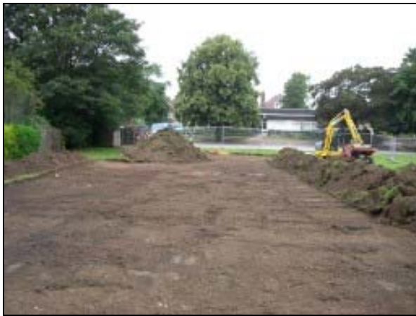
Plate 3: View north across new hard court
