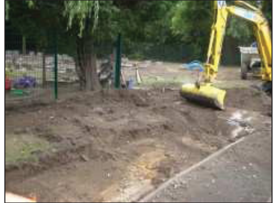
Plate 2: View NNW of ground clearance
