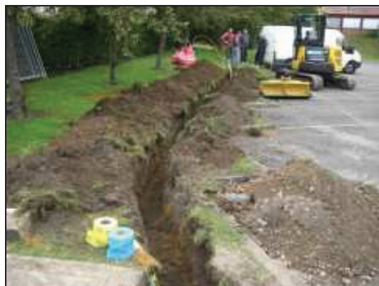
Plate 5: Middle section of service trench looking NNW
