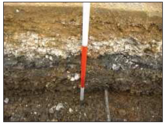
Plate 4: Make up of ground in service trench looking south west
