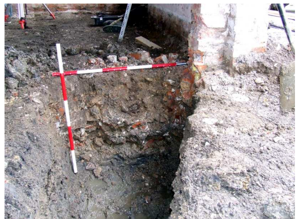
Plate 6: Internal wall foundation revealed at eastern side of entrance arches, facing E
