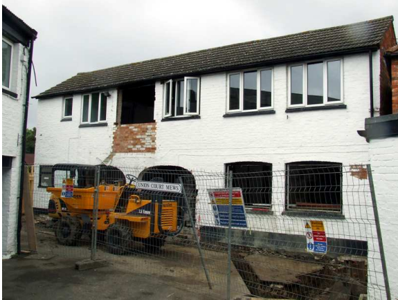
Plate 1: Southern elevation of conversion, facing NNW
