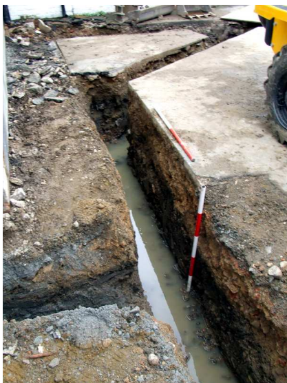
Plate 5: Drainage trench in courtyard, facing E
