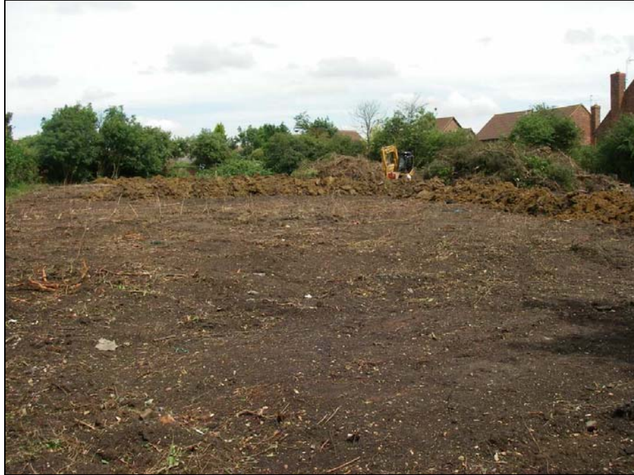
Plate 1: General view of site, looking north east
