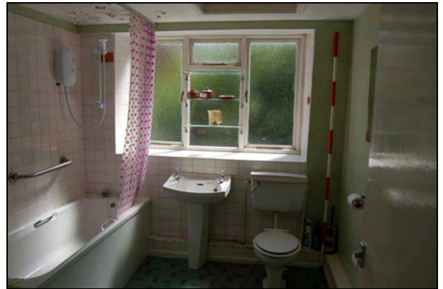
Plate 68: Room F11: south wall
