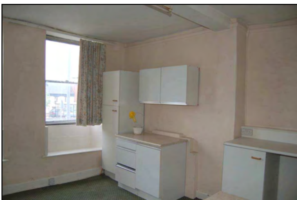
Plate 29: Room F2: southeast corner
