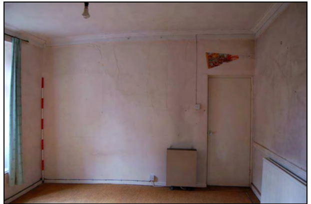
Plate 64: Room F8: west wall
