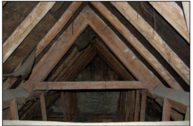
Plate 50: Attic looking south
