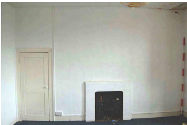
Plate 35: Room S1: north wall
