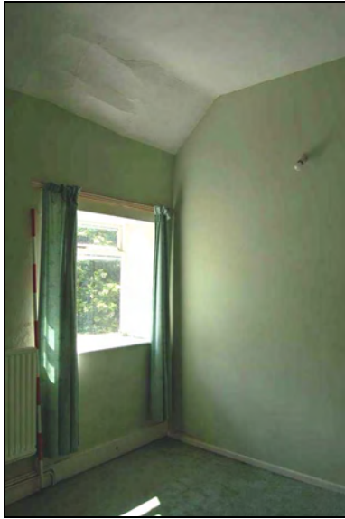
Plate 67: Room F10: southeast corner
