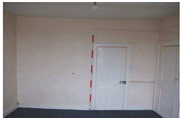
Plate 24: Room F1: west wall
