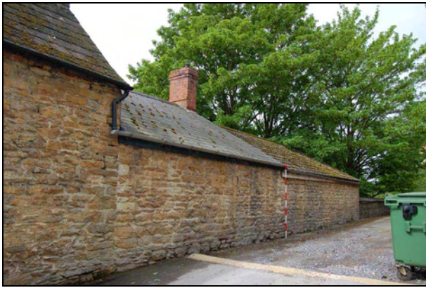
Plate 7: North elevation: Building 3
