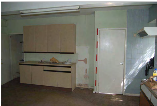
Plate 53: Room G8: east wall
