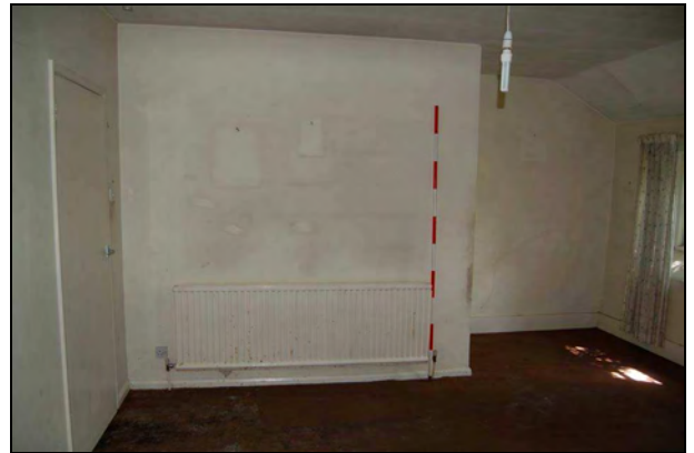
Plate 70: Room F12: east wall
