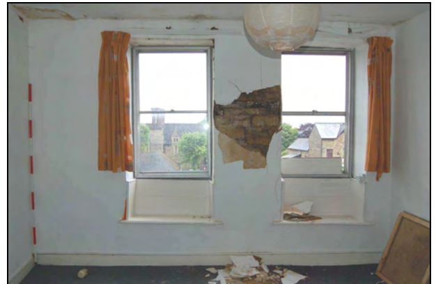
Plate 34: Room S1: east wall
