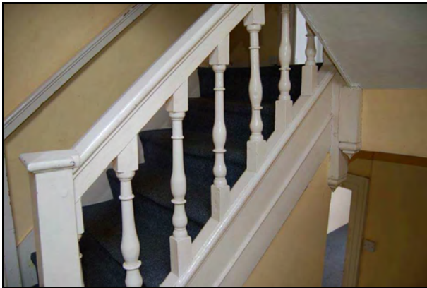
Plate 33: Room F7: stair detail
