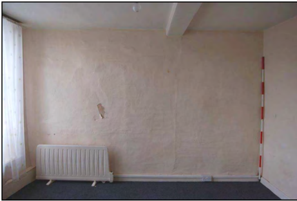
Plate 25: Room F1: south wall
