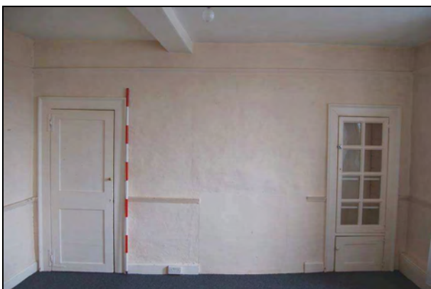
Plate 23: Room F1: north wall
