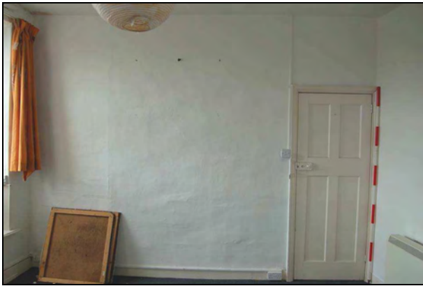
Plate 37: Room S1: south wall
