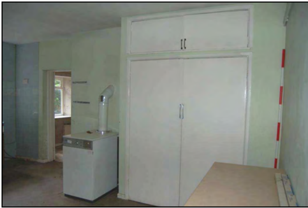
Plate 55: Room G8: west wall
