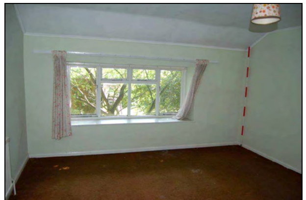
Plate 72: Room F13: south wall
