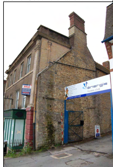
Plate 4: North elevation: Building 1
