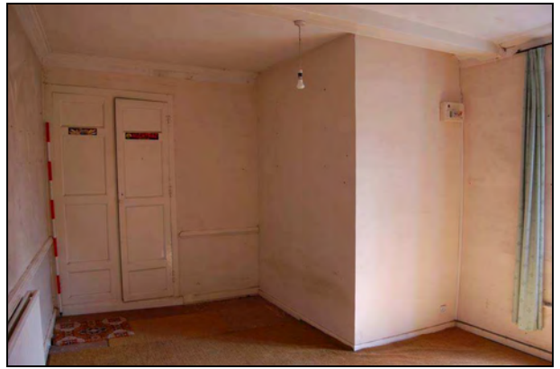
Plate 62: Room F8: east wall
