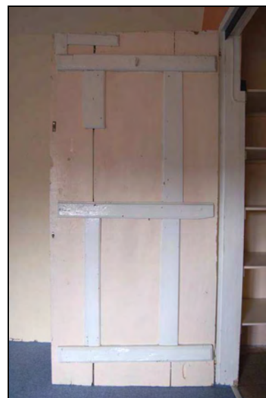
Plate 48: Room S4: cupboard door (internal)
