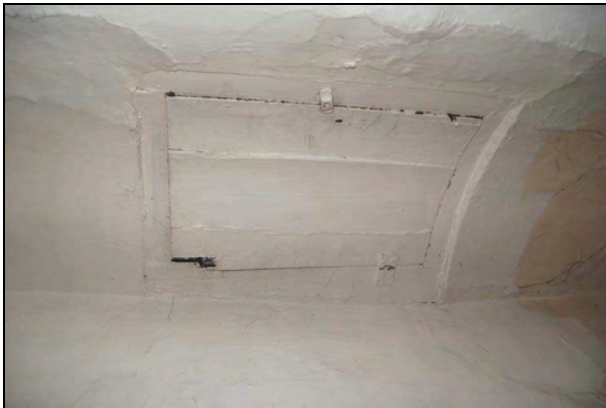
Plate 21: Room G4: fireplace ceiling with hatch
