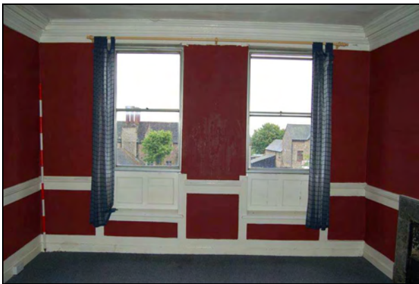
Plate 39: Room S2: east wall
