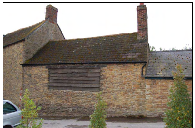
Plate 6: North elevation: Building 2
