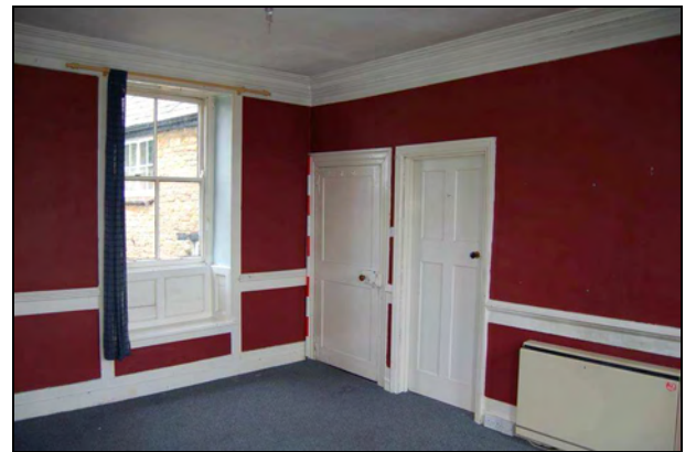
Plate 40: Room S2: northwest corner
