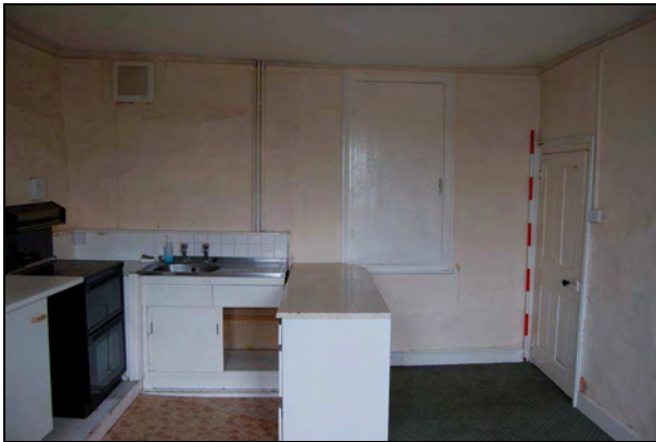
Plate 27: Room F2: west wall
