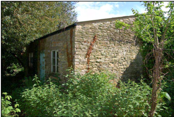
Plate 75: Shed: north & west elevations
