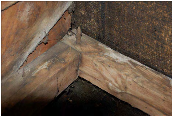
Plate 51: Attic: carpenters assembly mark
