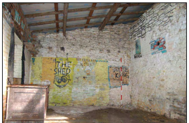
Plate 78: Shed: east wall
