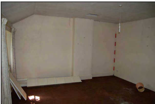
Plate 71: Room F12: west wall
