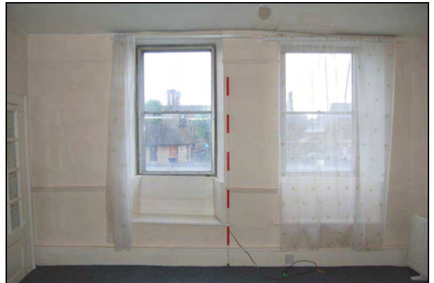
Plate 22: Room F1: east wall
