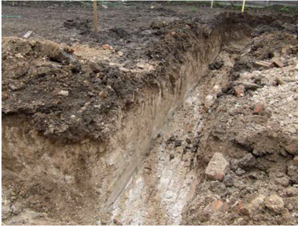
Plate 1: Southwest facing section of northeast footing
