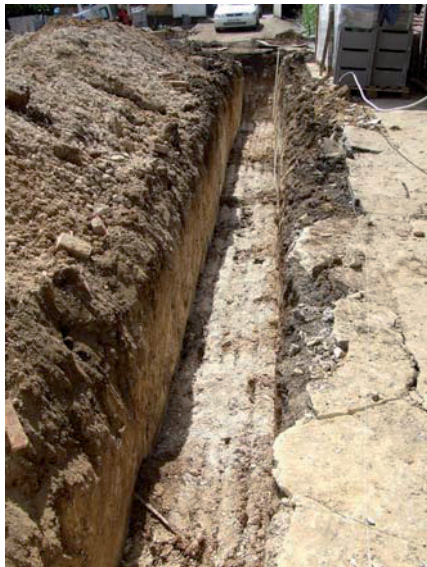
Plate 5: Northwest facing section of northwest footing
