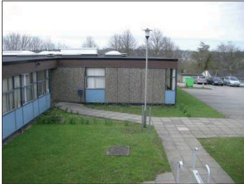
Plate 1: View looking west before work commenced on site
