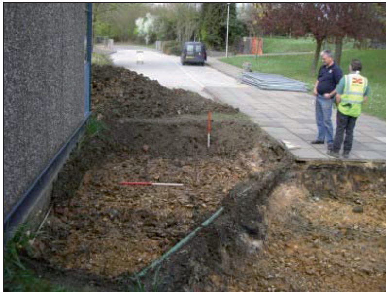
Plate 2: Western side of exposed area looking northwards
