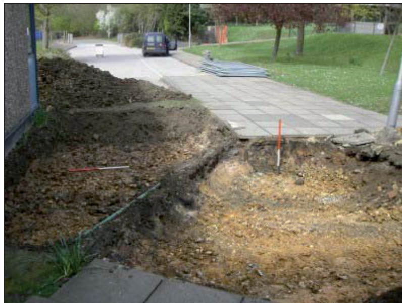
Plate 4: Area cleared of overburden looking north
