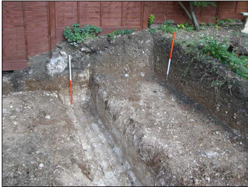
Plate 1: View of ground reduction and foundation trench, looking north (2x 1m scales)
