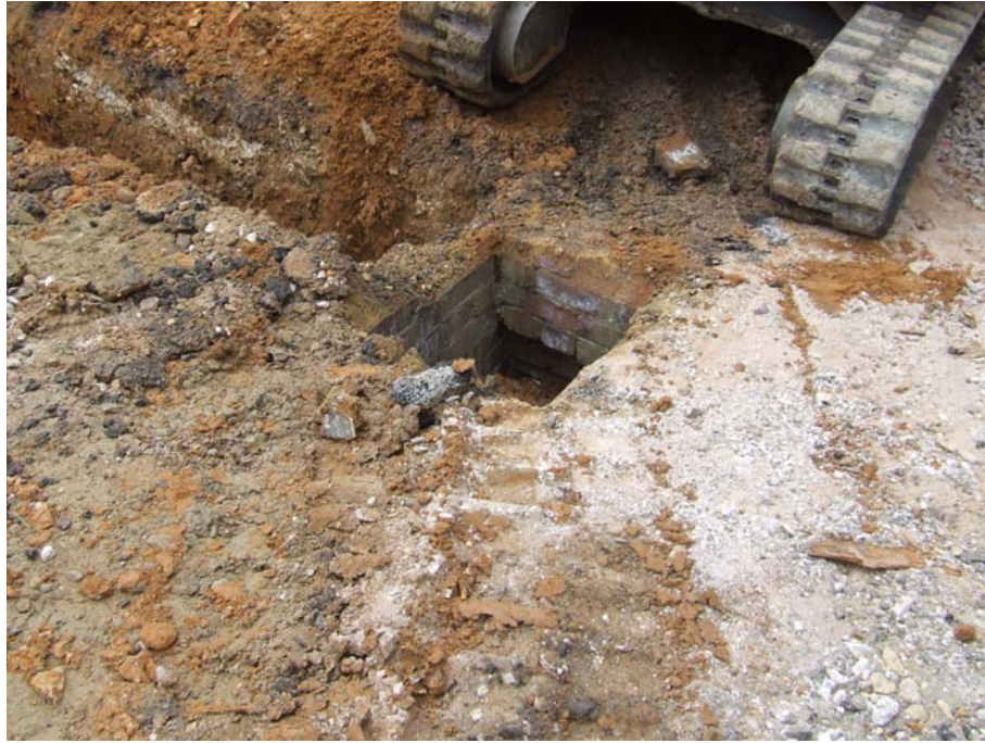
Plate 7: Drainage inspection chamber
