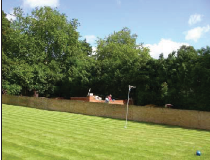
Plate 1: Setting of the new swimming pool
