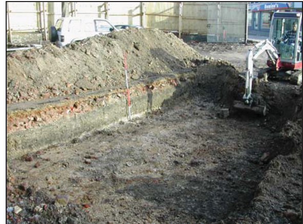
Plate 2: View east across trench with machining underway (Scale = 2m)
