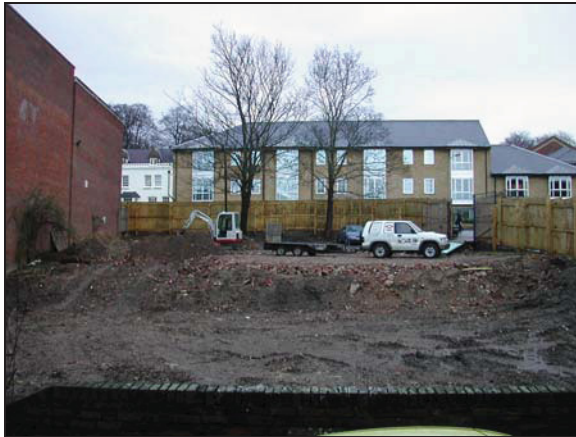
Plate 1: View northwards across the site
