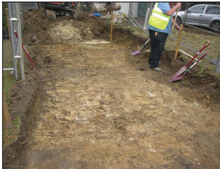
Plate 3: The access corridor as stripped, looking north.
