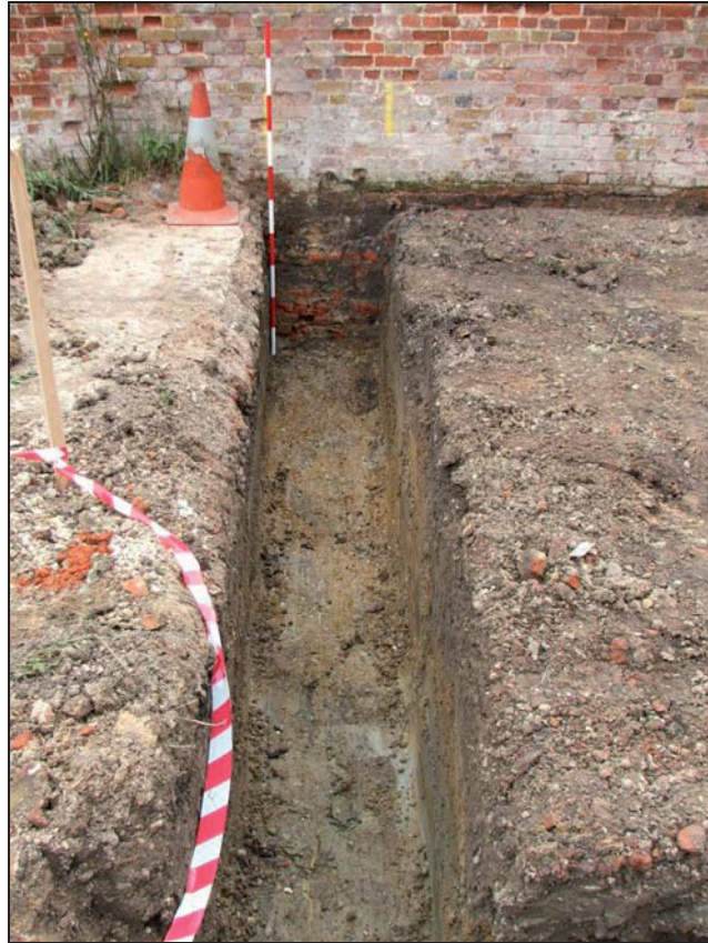
Plate 12: North footing trench: footings of east wall
