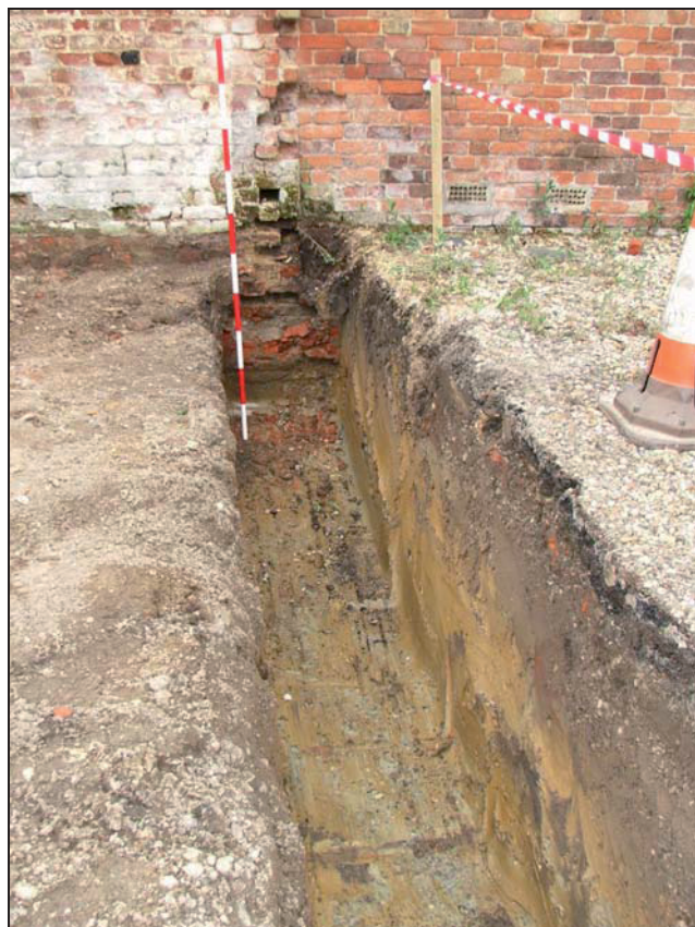
Plate 13: West footing trench: footings of south wall
