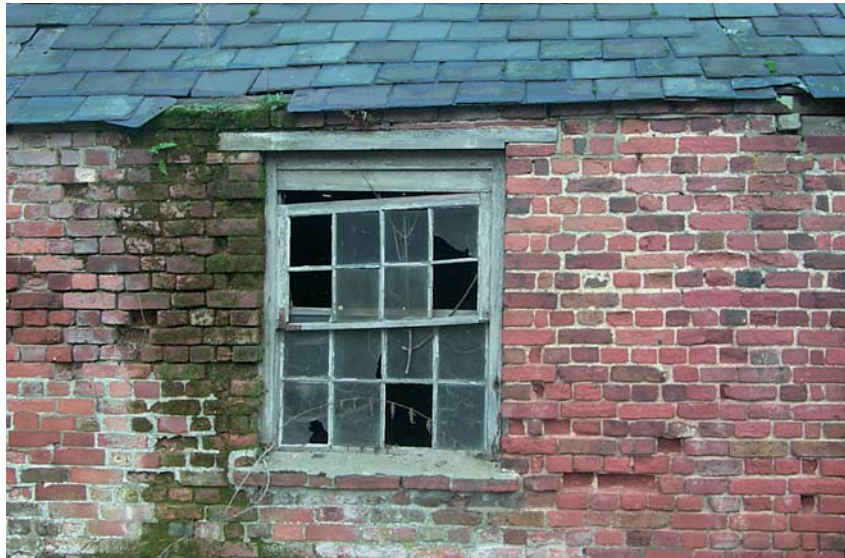
Plate 7: West elevation, window
