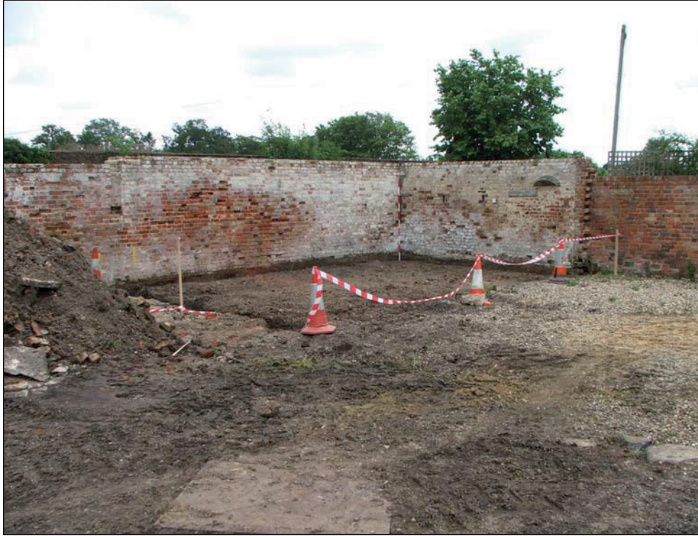
Plate 10: Site of new garage, after completion of groundworks
