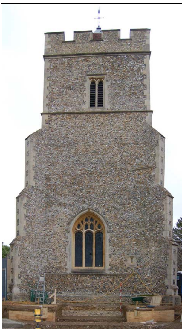
Plate 40: West elevation of tower
