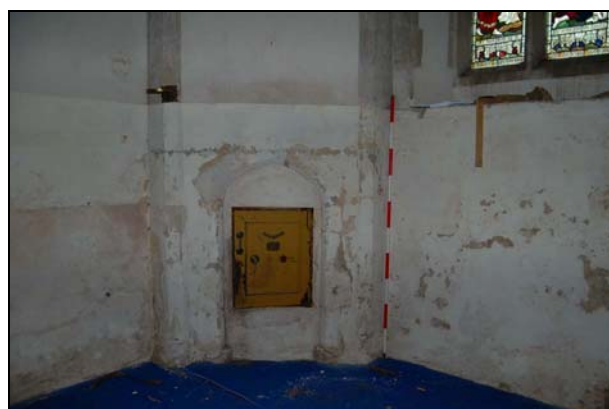
Plate 43: Blocked door in the southwest corner
