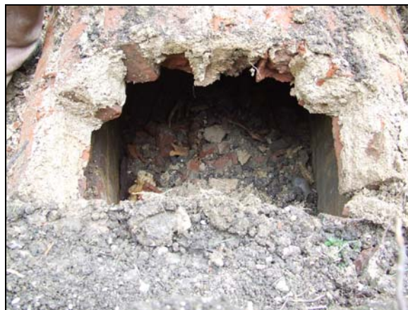
Plate 15: Burial HB 28, roof of brick vault
