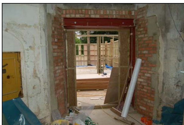
Plate 48: New opening in the west wall
