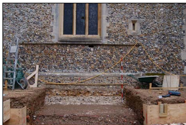
Plate 47: External ground reduction
