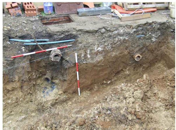
Plate 6: Ceramic drains cut into (102), facing SSW
