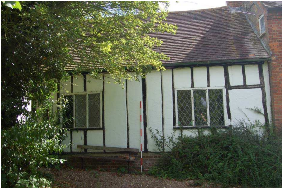
Plate 7: Building 2: west elevation
