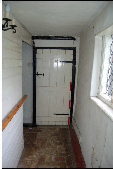
Plate 25: Room G4: looking south
