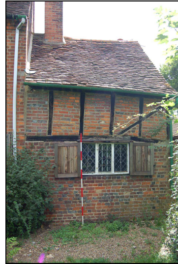
Plate 8: Building 3: west elevation
