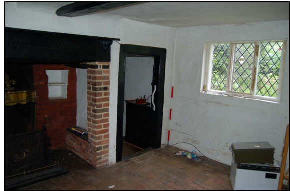
Plate 20: Room G3: southwest corner
