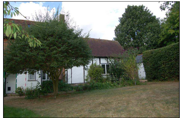
Plate 4: Building 2: east elevation
