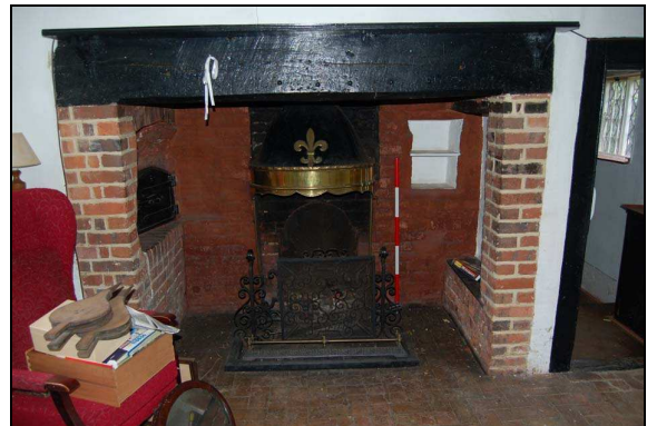
Plate 22: Room G3: fireplace detail
