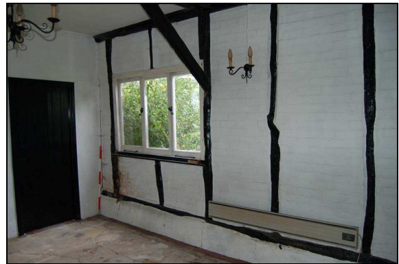
Plate 34: Room G6: southwest corner
