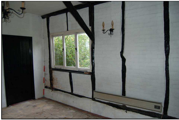
Plate 31: Room G6: northeast corner
