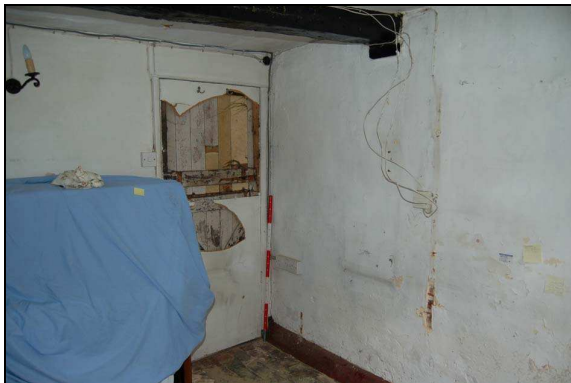
Plate 27: Room G5: northwest corner
