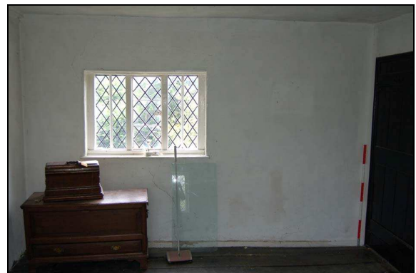
Plate 42: Room F2: west wall
