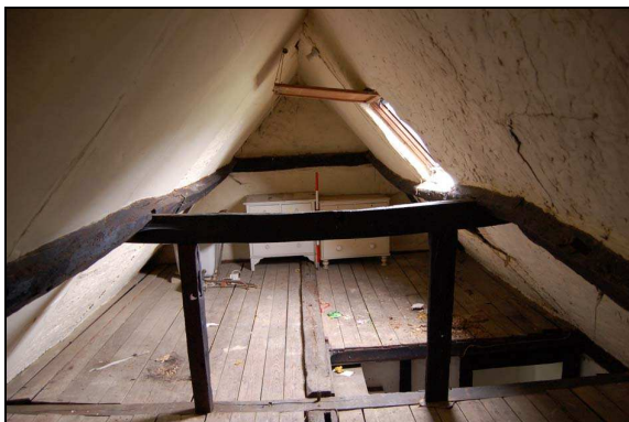
Plate 47: Room S1: looking north
