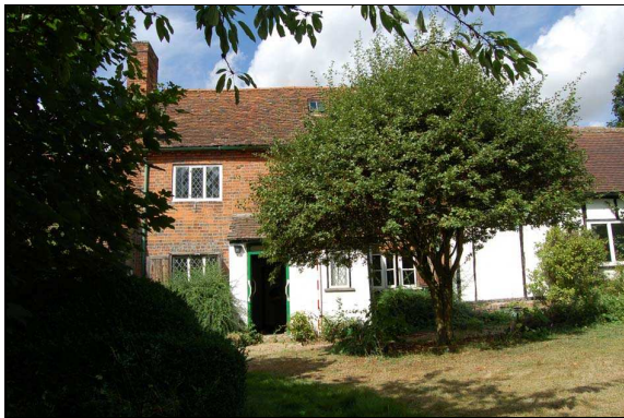
Plate 3: Building 1: east elevation
