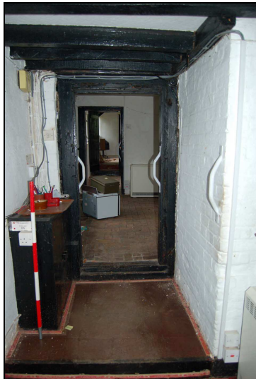
Plate 15: Room G2: northwest corner
