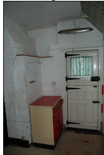
Plate 10: Room G1: northwest corner
