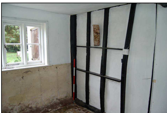
Plate 29: Room G5: southeast corner
