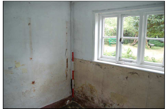
Plate 26: Room G5: northeast corner
