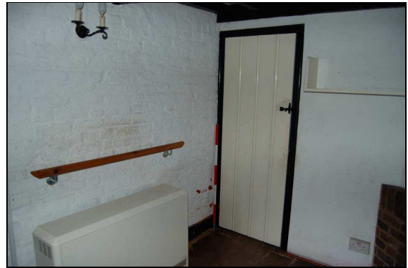
Plate 14: Room G2: northeast corner
