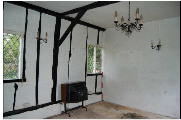
Plate 32: Room G6: northeast corner
