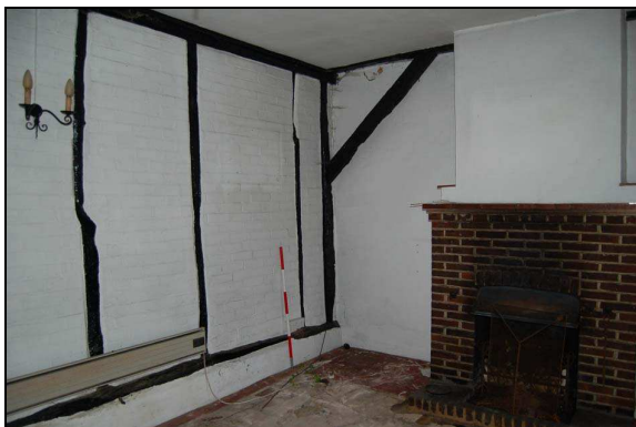
Plate 35: Room G6: southeast corner
