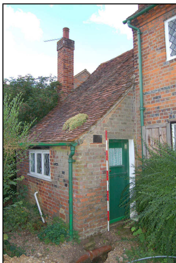
Plate 5: Building 3: east elevation
