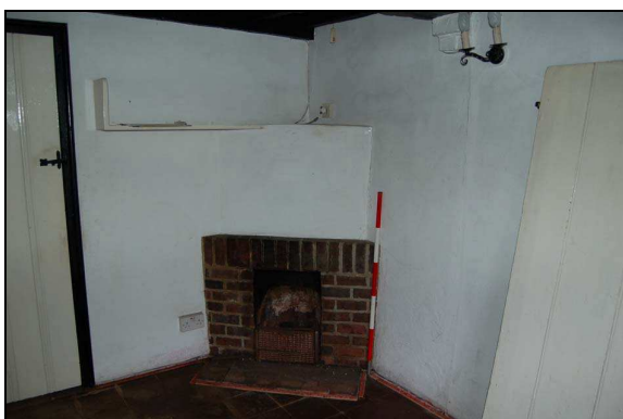
Plate 17: Room G2: southeast corner
