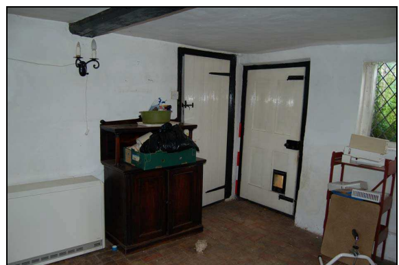
Plate 18: Room G3: northeast corner
