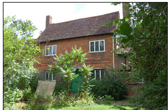
Plate 6: Building 1: west elevation
