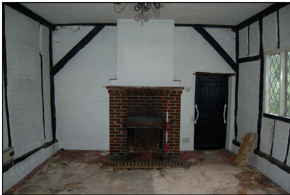
Plate 33: Room G6: south wall
