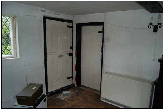
Plate 19: Room G3: northwest corner
