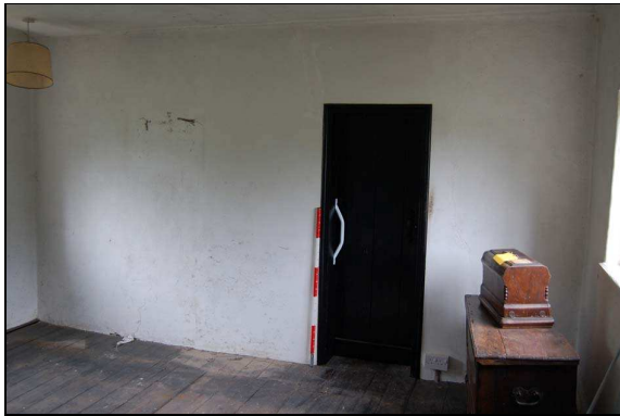
Plate 43: Room F2: south wall
