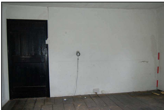
Plate 41: Room F2: north wall
