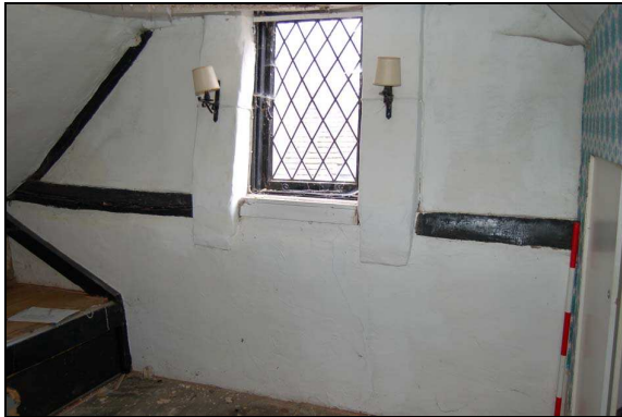
Plate 39: Room F1: south wall
