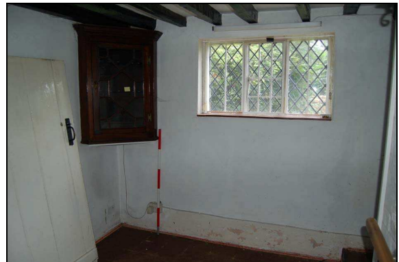
Plate 16: Room G2: southwest corner
