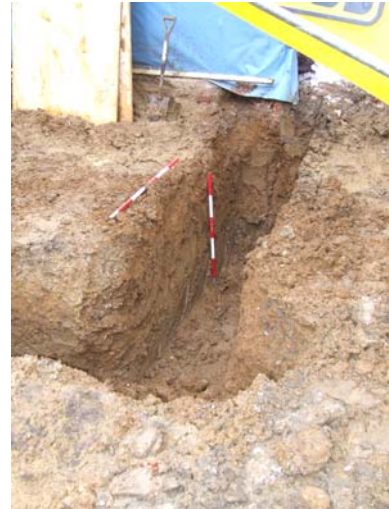
Plate 2: Detail of western part of footing, facing NW
