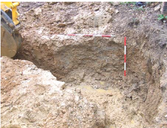
Plate 3: Natural feature at SW of footing, facing S
