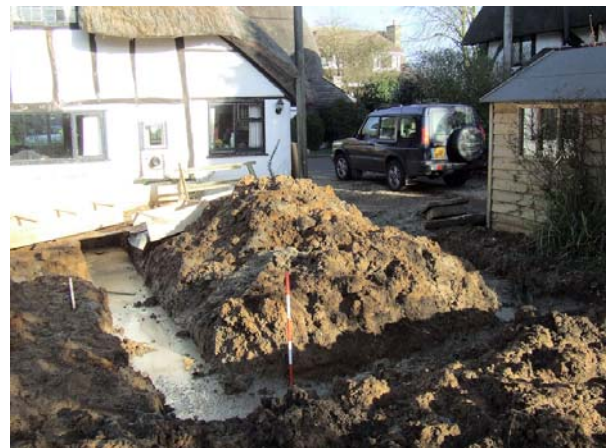
Plate 4: Eastern half of footings, facing NE
