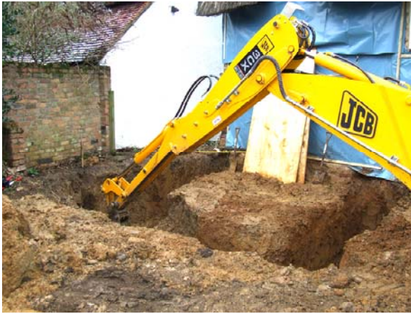
Plate 1: Excavation of western half of footings, facing NW
