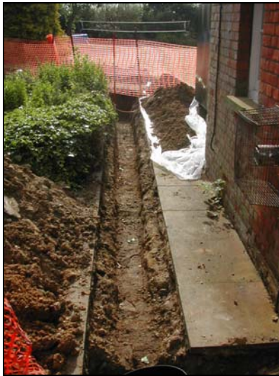
Plate 3: Service trench outside house, looking east 30/06/06
