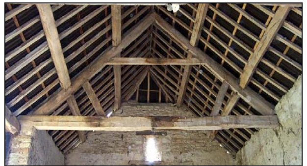
Plate 10: Southern roof truss
