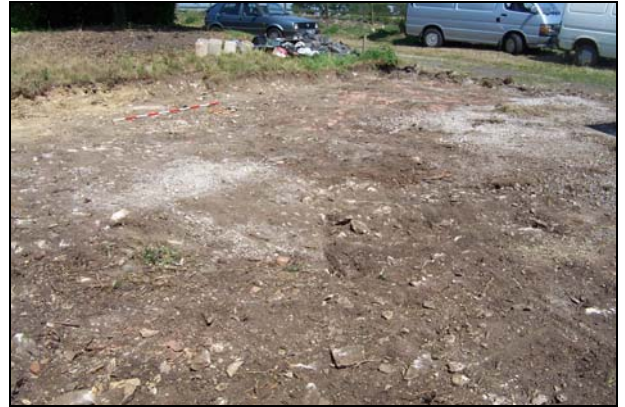
Plate 14: External ground reduction looking north
