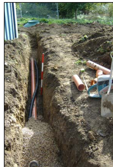
Plate 18: Drainage trench looking southeast
