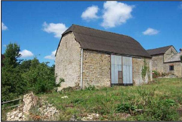
Plate 1: South & east elevations
