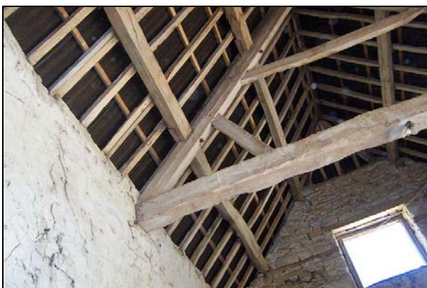
Plate 11: Face halved joints and metal bolts
