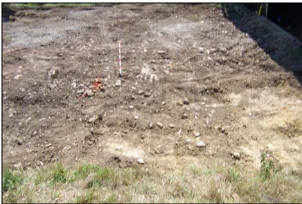
Plate 15: External ground reduction looking south
