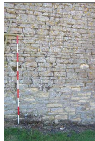
Plate 12: North elevation stonework detail
