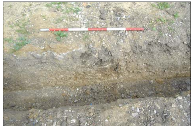
Plate 16: Northern garage footing trench looking north
