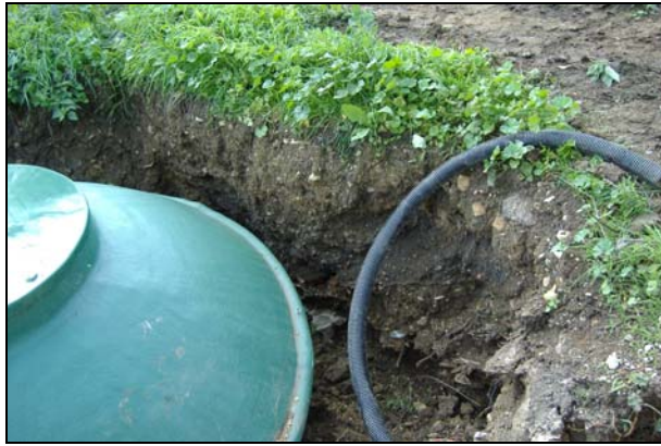
Plate 19: East facing section of the septic tank
