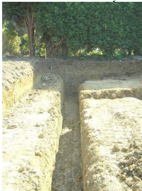
Plate 2: General view of the footing trench Plot 1
