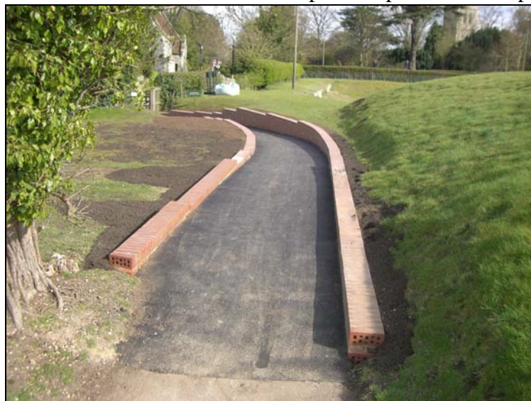
Plate 2: View west looking down slope of new footpath
