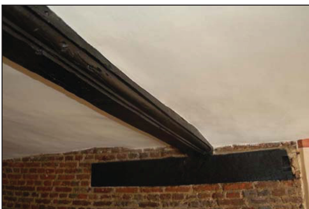
Plate 23: Room G8: moulding detail
