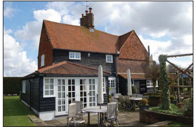
Plate 2: West elevation from the NW
