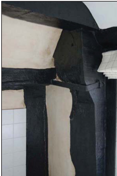
Plate 47: Room F6: south east corner detail
