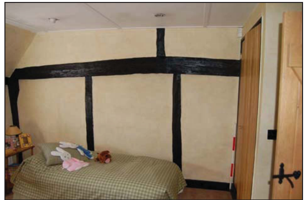
Plate 34: Room F3: west wall
