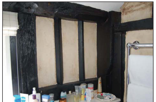
Plate 48: Room F6: former window in east wall
