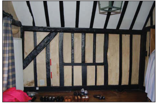
Plate 44: Room F5: east wall
