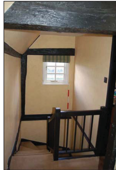
Plate 28: Room F1: east wall
