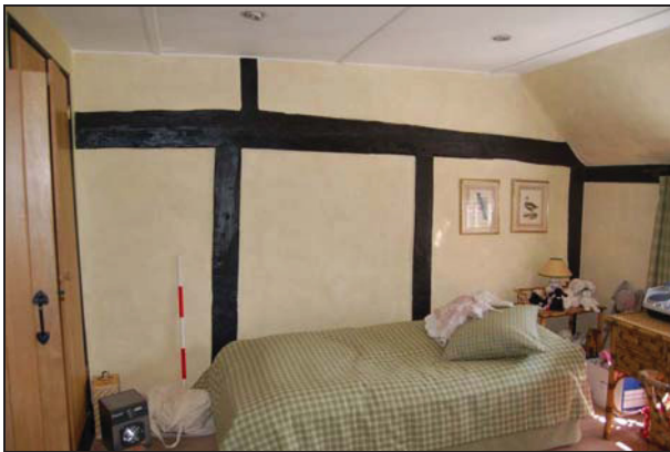
Plate 33: Room F3: east wall
