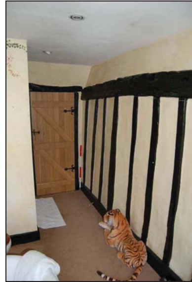
Plate 38: Room F4: close studding in north wall
