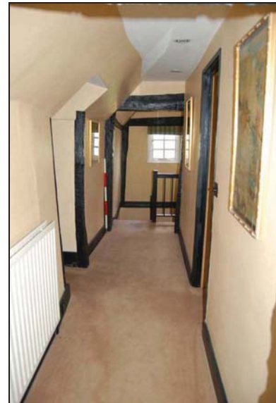
Plate 30: Room F1: looking east
