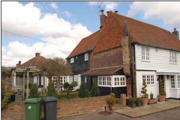
Plate 3: West elevation from the SW
