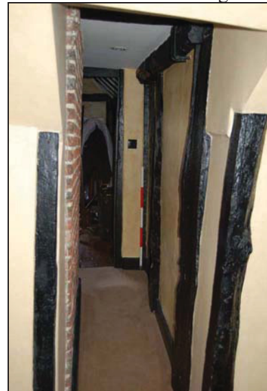
Plate 40: Passage to Room F5
