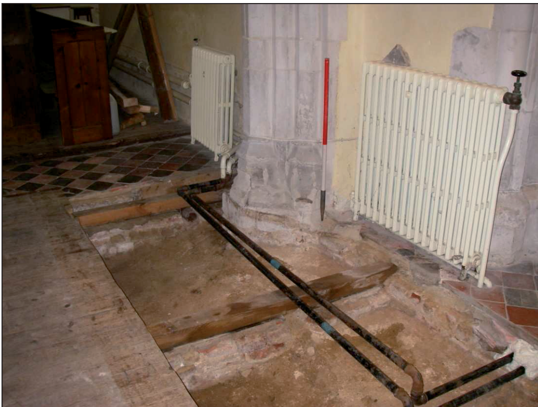
Plate 6: The raised floor support beams in the chancel
