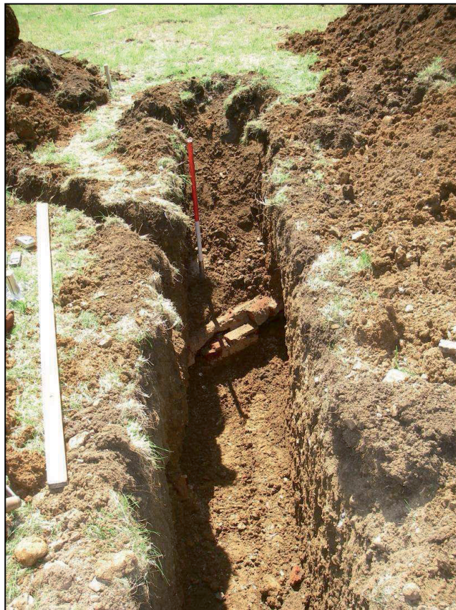
Plate 4: The sewer trench and part of the brick vault
