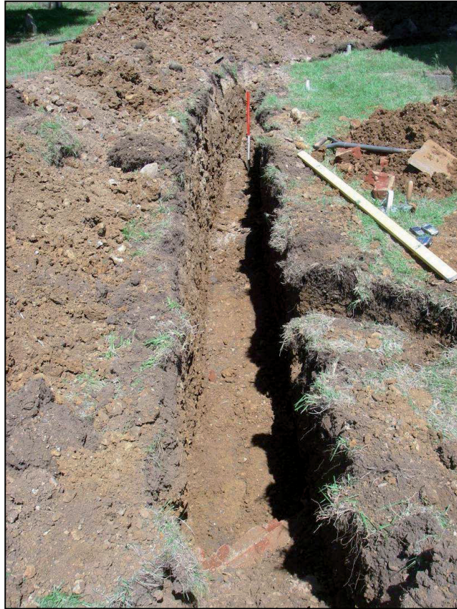
Plate 3: The sewer trench looking north east
