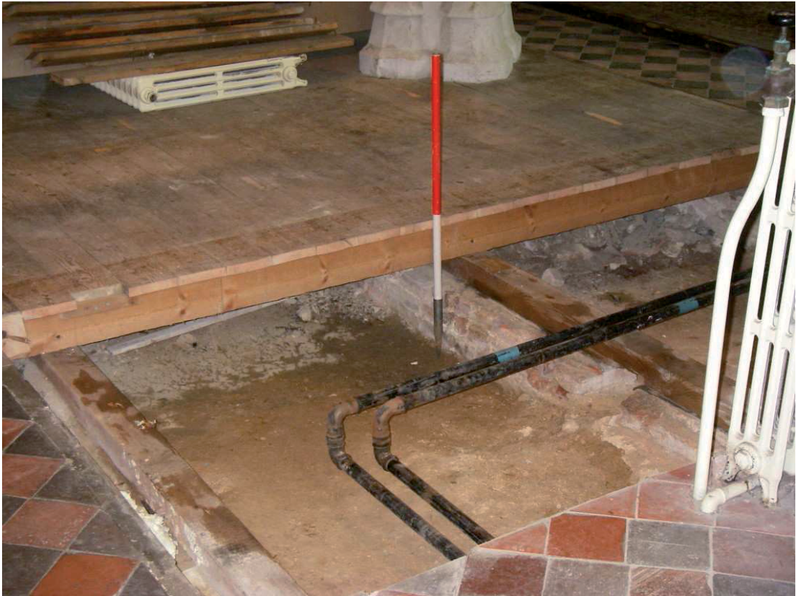
Plate 7: Detail of the void under the raised floor
