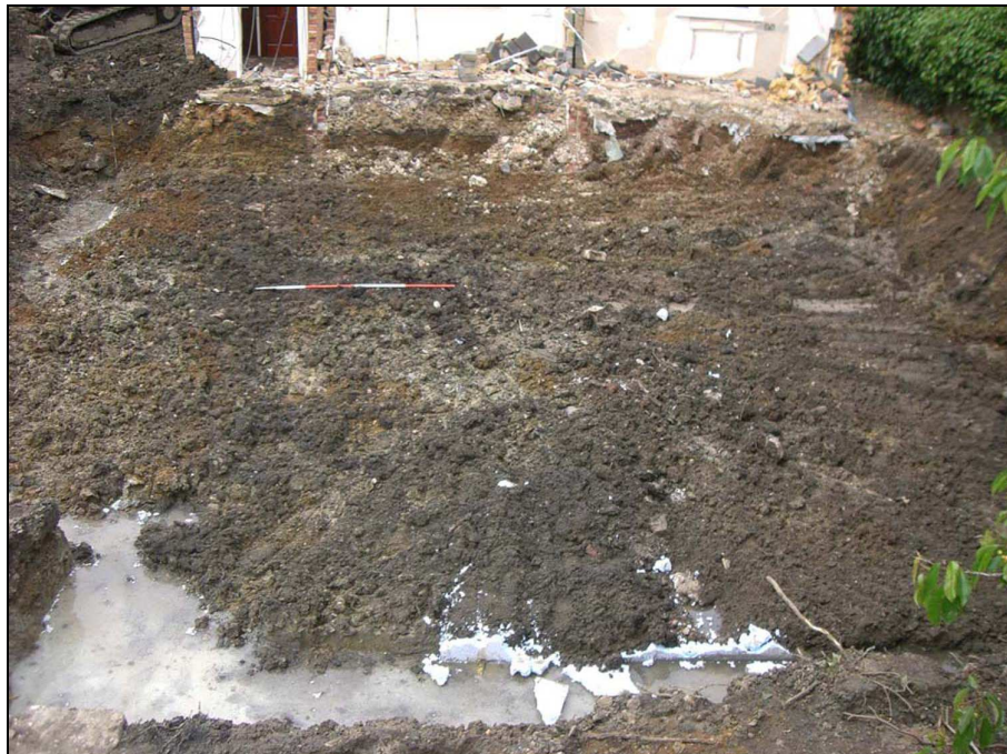
Plate. 2: Soil horizons at the south end of the site
