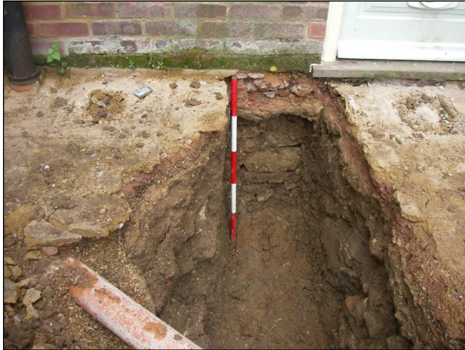
Plate 3: Footings for the rear wall of 110 High Street
