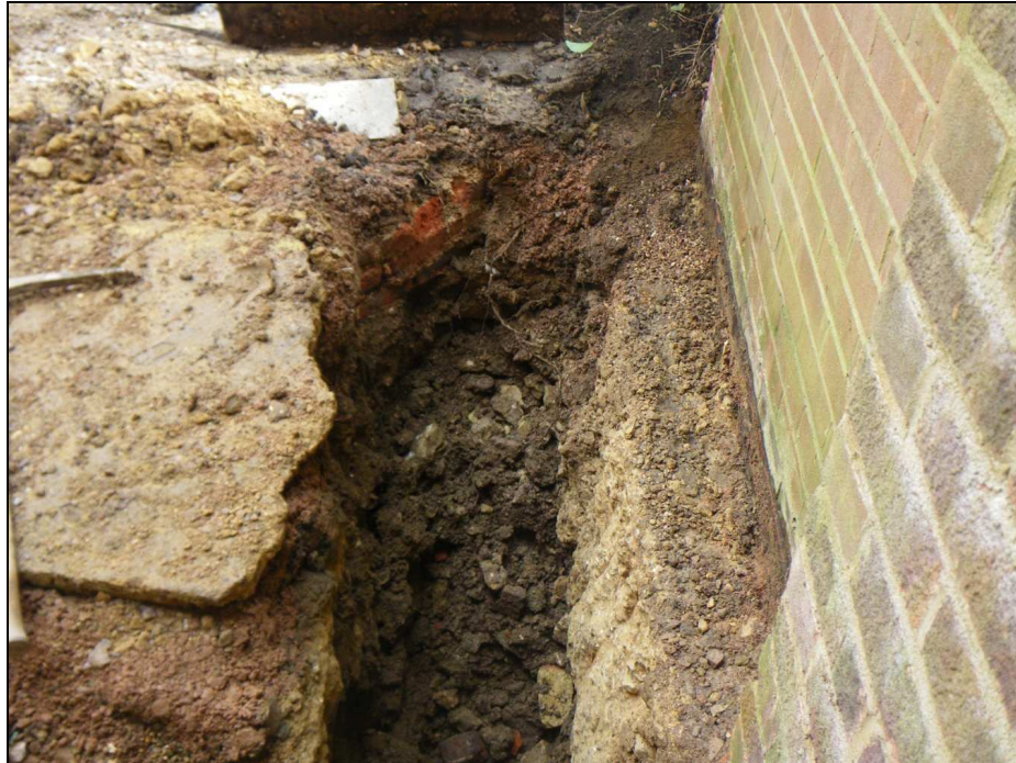
Plate 5: Brick wall at the junction of Trenches A & B
