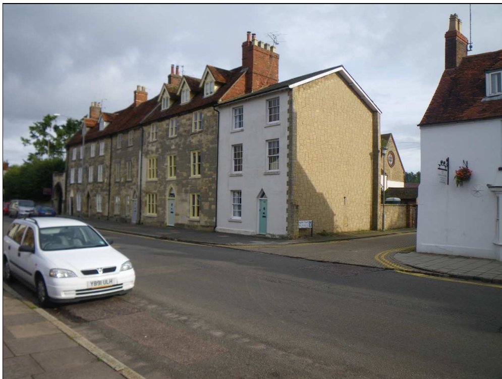
Plate 2: 108 to 114 High Street (note the partial demolition of 108 to create the new access road)
