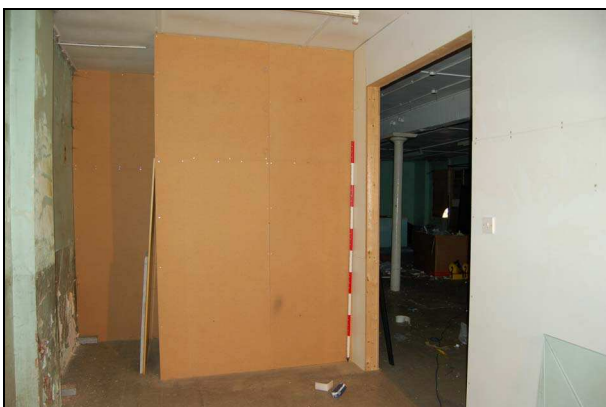
Plate 23: Room G5: east wall
