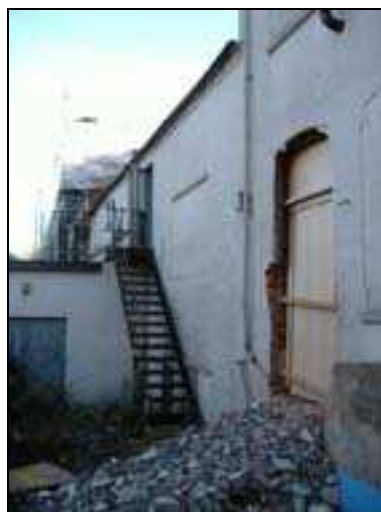
Plate 41: Inner yard south
