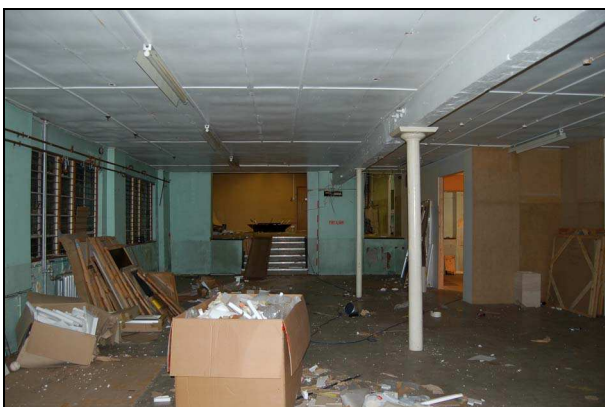
Plate 17: Room G3: looking west
