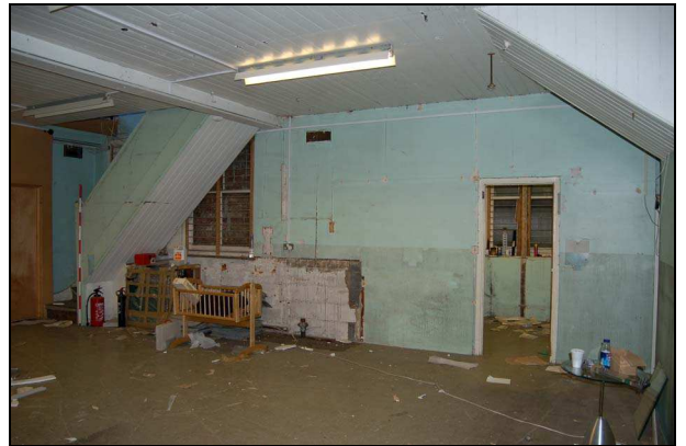
Plate 14: Room G2: north wall
