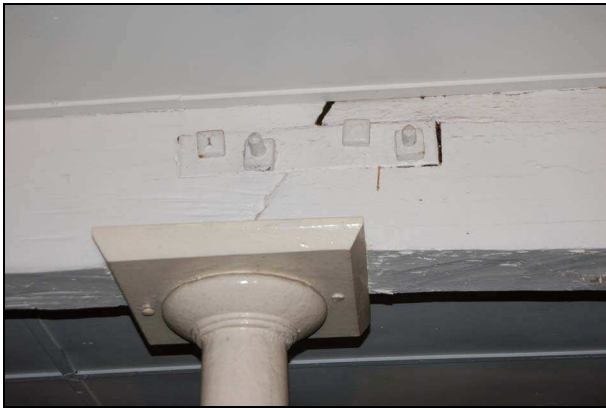
Plate 19: Room G3: column & scarf joint detail
