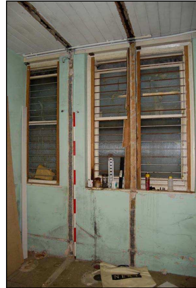
Plate 20: Room G4: north wall
