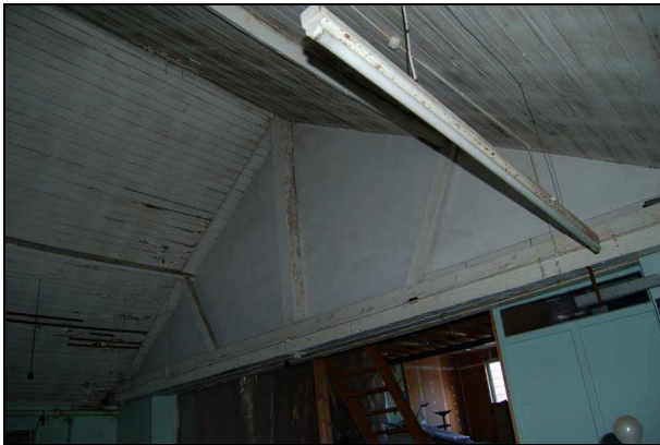
Plate 39: Room F2: roof truss
