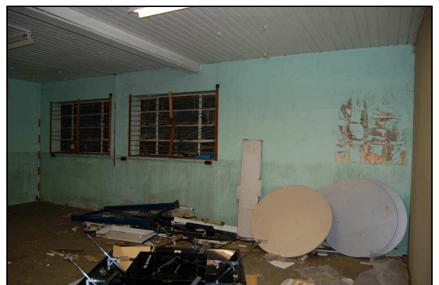
Plate 12: Room G2: south wall
