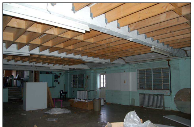
Plate 36: F2: north wall
