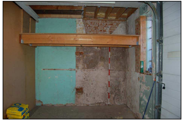
Plate 8: Room G1: south wall
