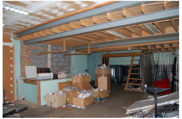
Plate 32: F1: north wall
