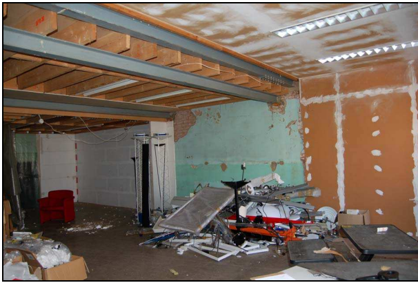
Plate 31: F1: south wall
