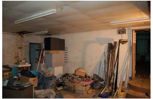
Plate 28: Room G6: south wall
