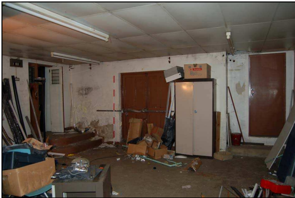
Plate 27: Room G6: west wall
