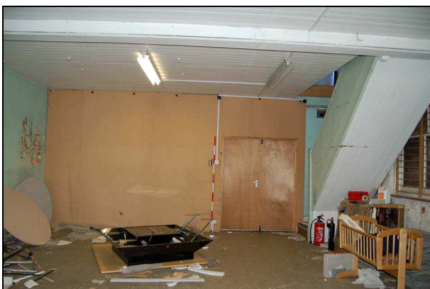
Plate 11: Room G2: west wall
