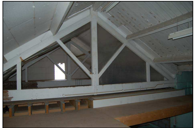
Plate 34: F1: roof truss
