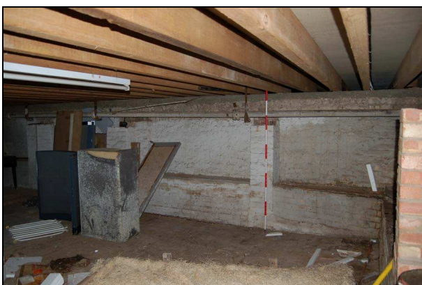
Plate 5: Room C1: west wall
