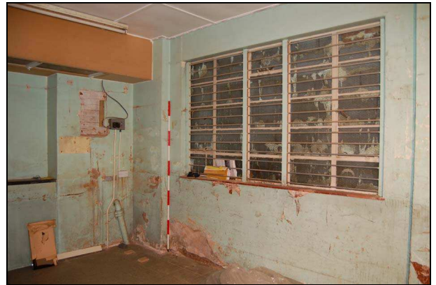
Plate 22: Room G5: northwest corner
