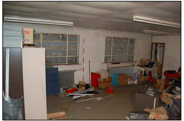
Plate 26: Room G6: north wall
