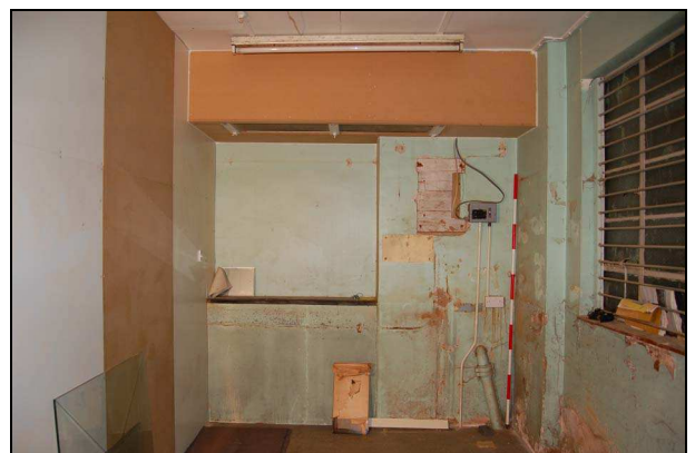
Plate 24: Room G5: west wall
