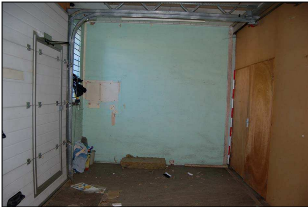
Plate 9: Room G1: north wall
