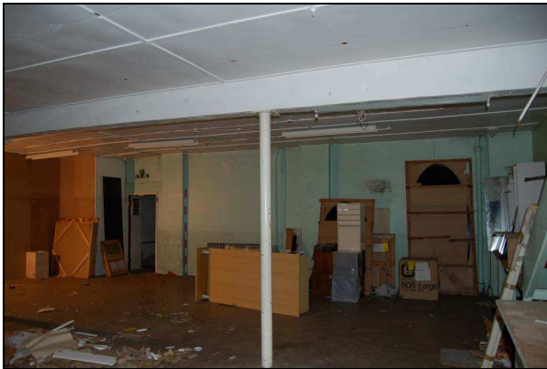
Plate 15: Room G3: north wall
