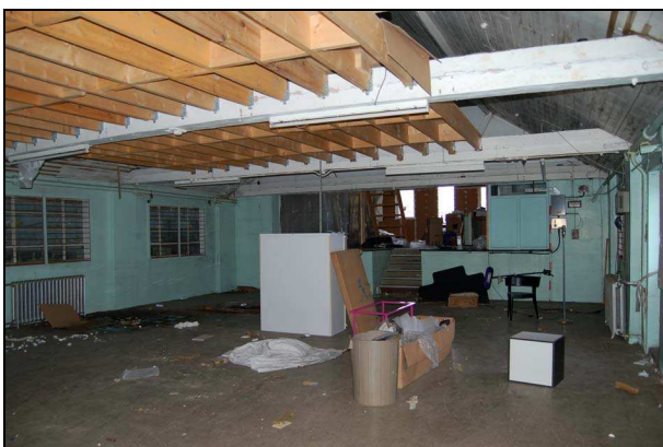
Plate 35: F2: looking southwest
