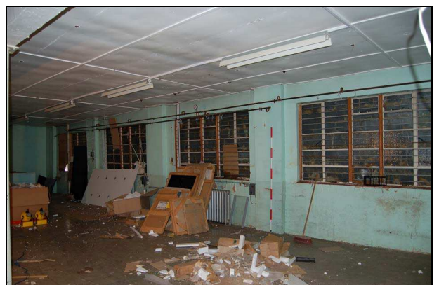
Plate 18: Room G3: south wall
