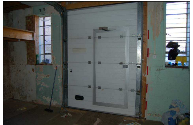
Plate 10: Room G1: west wall
