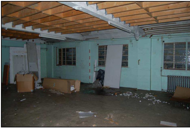
Plate 37: Room F2: southeast corner
