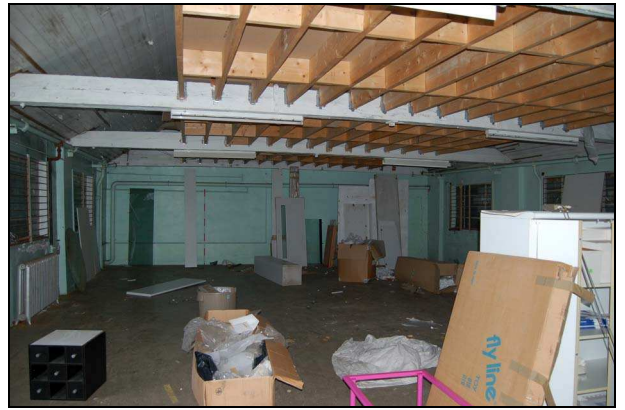
Plate 38: Room F2: looking east
