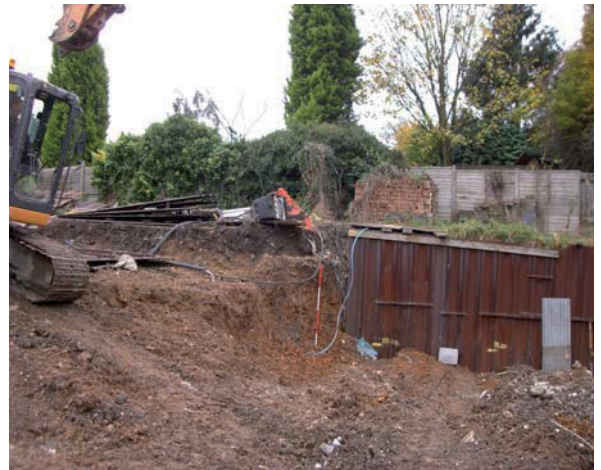
Plate 4: View looking north to north end of site
