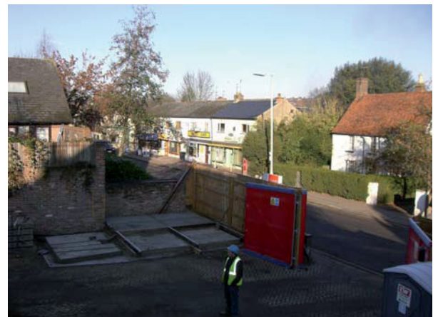
Plate 6: Entrance to site from Akeman St/HighSt
