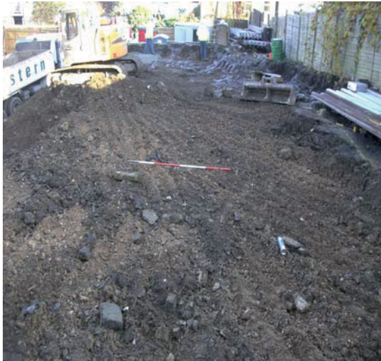
Plate 1: Natural gravely clay at southern end of site
