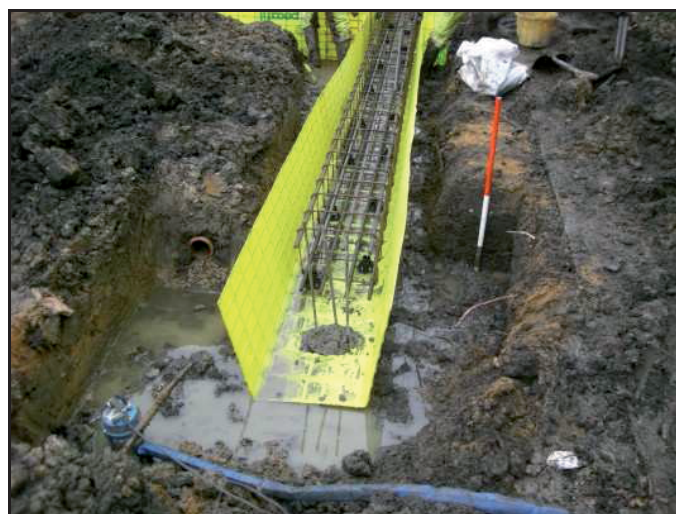
Plate 3: Detail of the foundation construction cutting through buried soil and subsoil
