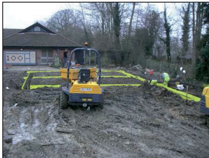
Plate 2: Construction of the ring beam foundations.
