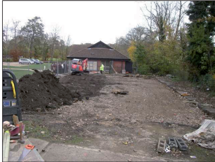
Plate 1: Footprint of the drama block, looking east, showing overburden stripping in progress.
