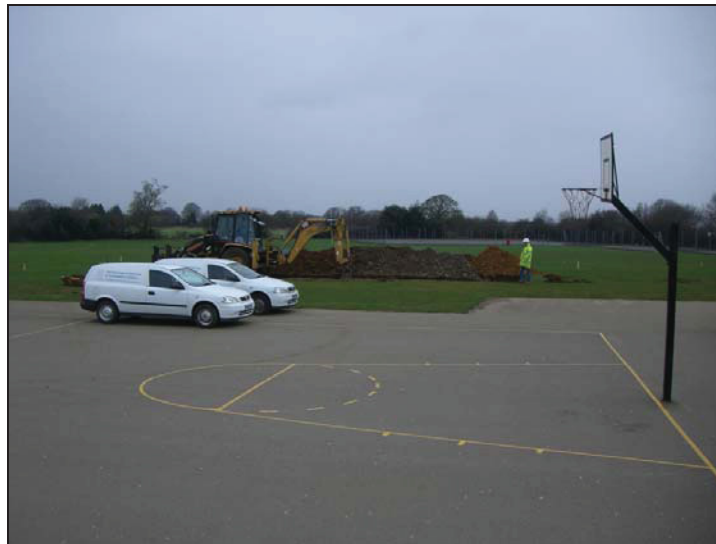
Plate 1: Machining trench, facing west
