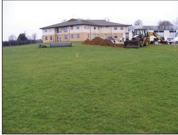
Plate 2: General view, facing northeast
