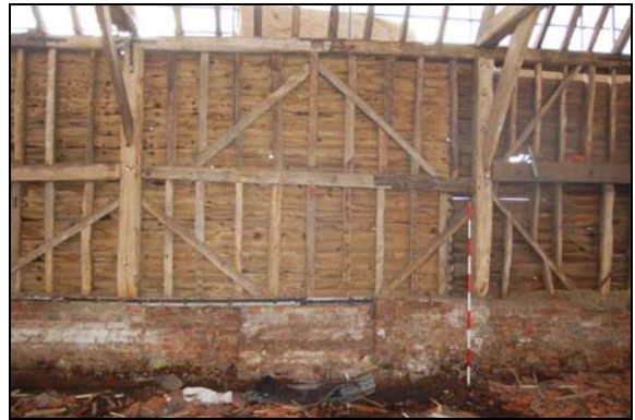
Plate 8: South wall: Bay 3
