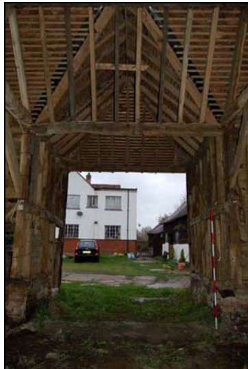
Plate 15: North wall: Bay 3
