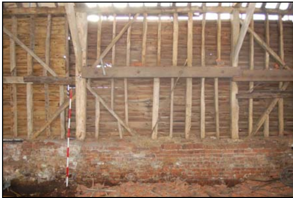
Plate 7: South wall: Bay 2
