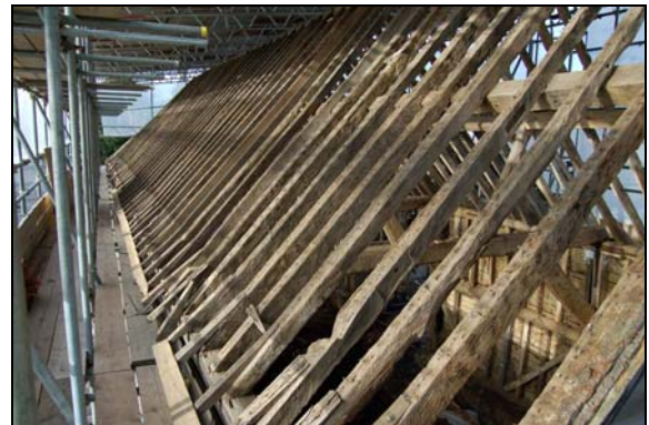
Plate 22: South side of the stripped roof
