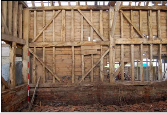
Plate 13: North wall: Bay 1
