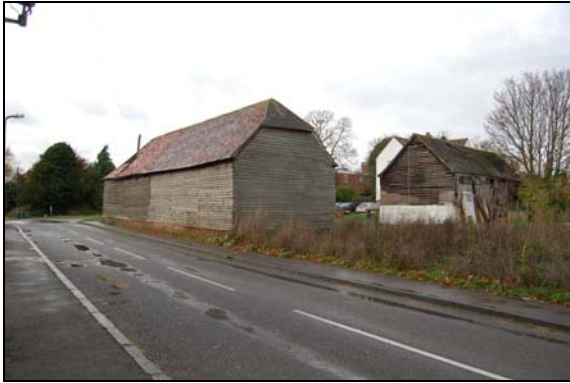
Plate 1: South & east elevations
