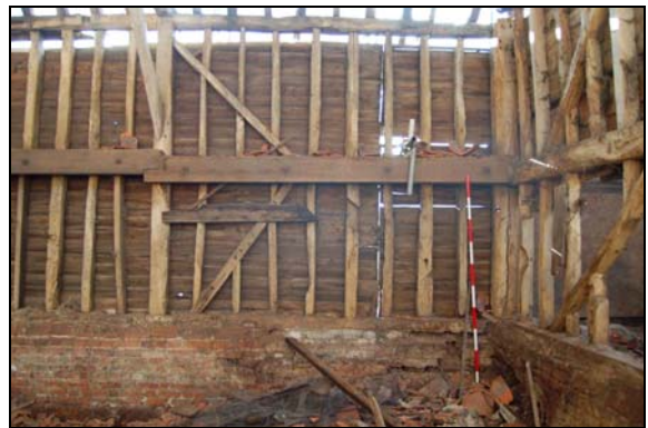
Plate 6: South wall: Bay 1
