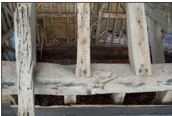
Plate 23: Carpenters assembly marks on a common rafter
