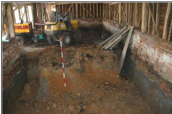
Plate 5: General ground reduction, looking east, 2m scale
