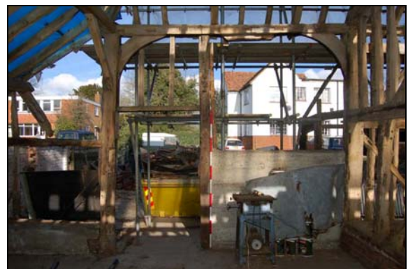
Plate 24: Western extension: north wall
