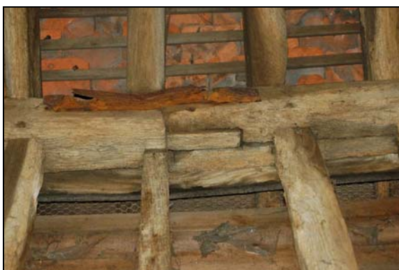
Plate 11: Bridled scarf joint in Bay 1
