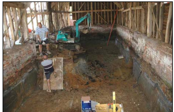
Plate 6: General ground reduction, looking east, 2m scale
