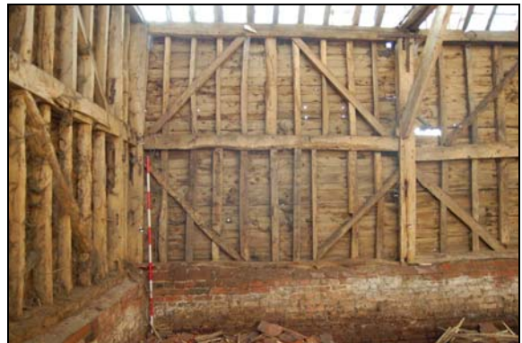
Plate 10: South wall: Bay 5
