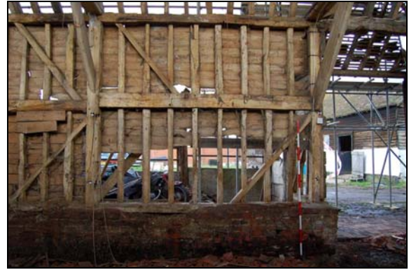
Plate 14: North wall: Bay 2
