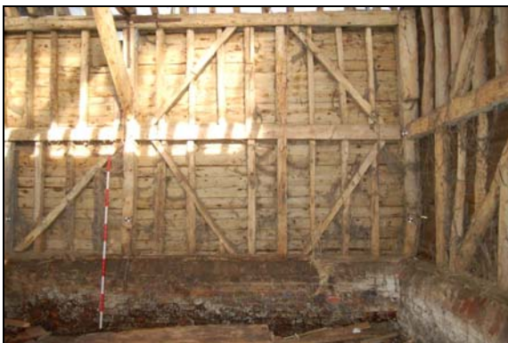
Plate 17: North wall: Bay 5
