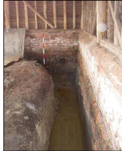
Plate 2: Underpinning trench, looking east, 2m scale
