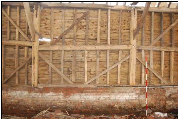
Plate 9: South wall: Bay 4
