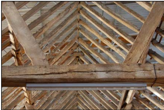
Plate 21: Carpenter's assembly marks
