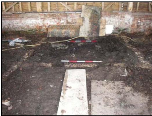
Plate 3: Brick footings, looking south, 2x 1m scale
