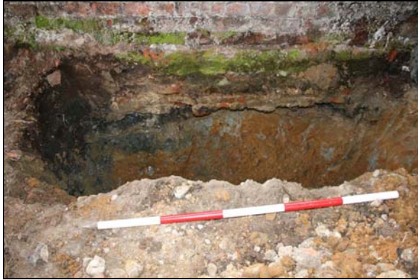
Plate 1: Underpinning pit 1, looking north, 1m scale
