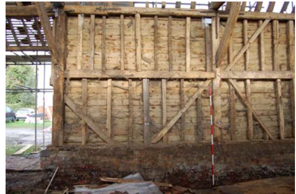
Plate 16: North wall: Bay 4
