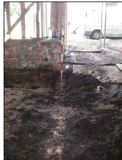
Plate 4: Brick footings, looking north, 1m scale
