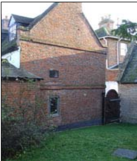
Plate 5: South east corner of garden, view to south east
