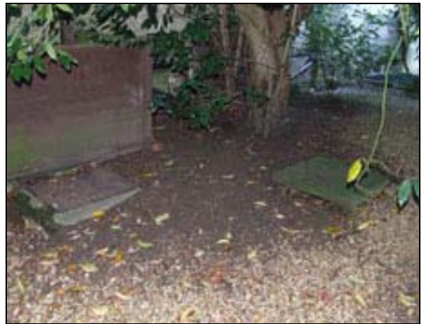
Plate 4: Drain covers on NE corner view to south west
