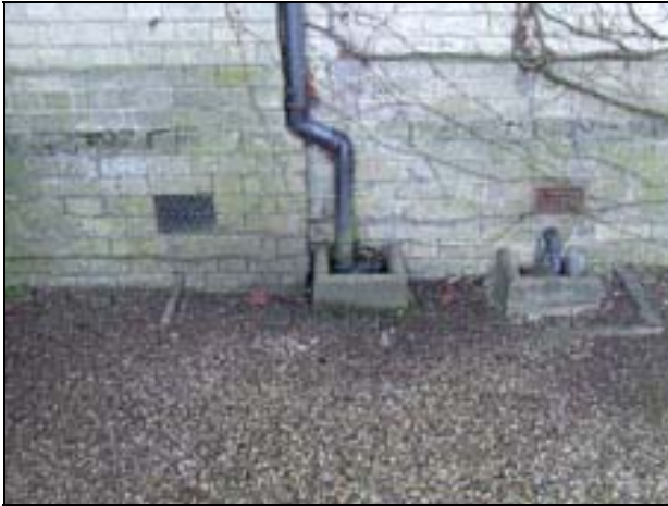
Plate 7: Pipes out of north side of building
