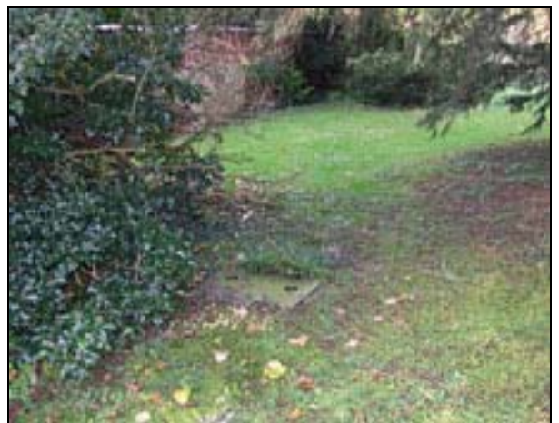
Plate 6: Drain on west of property, view to north west
