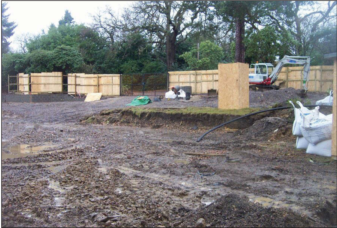
Plate 3: View of the central part of the site, looking south
