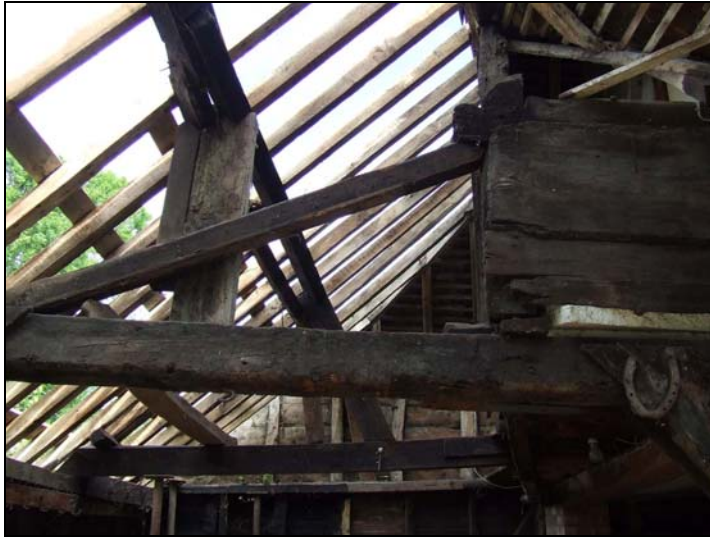
Plate 10: Truss 1 looking north
