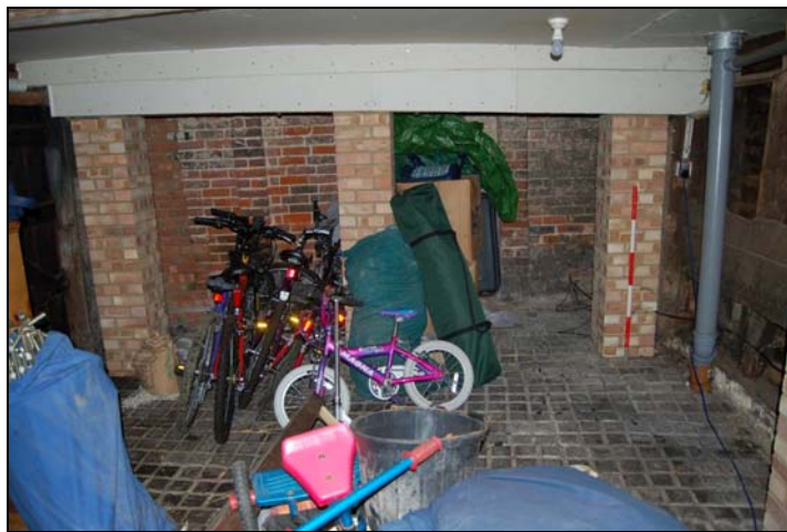
Plate 5: East wall of former stable
