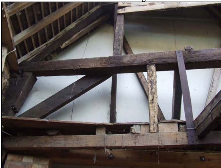
Plate 12: Northern end of roof truss at barn junction
