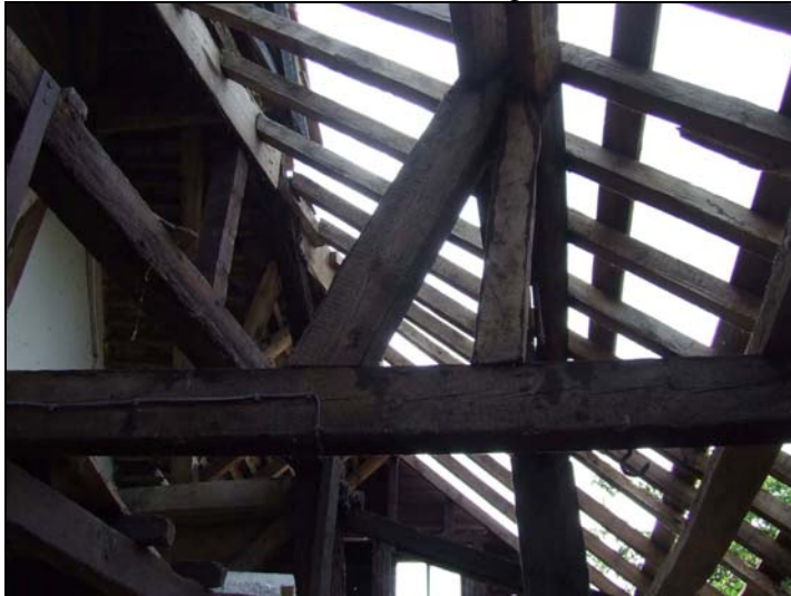
Plate 11: Truss 1 looking south
