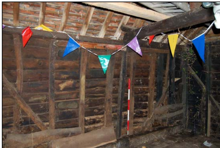
Plate 9: Northwest corner of western end of barn
