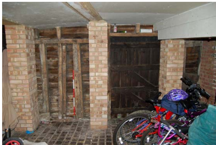
Plate 6: North wall of former stable
