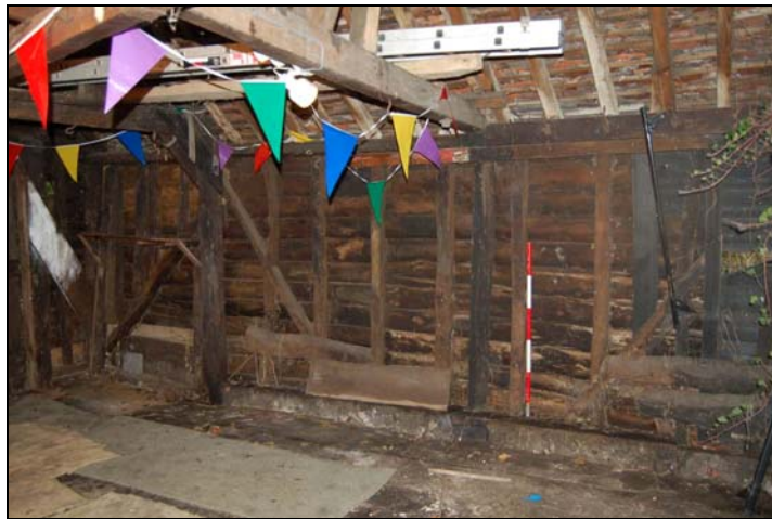
Plate 8: Southwest corner of western end of barn
