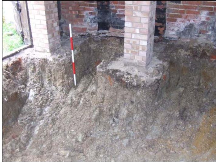
Plate 14: Northeast corner of the barn during ground reduction
