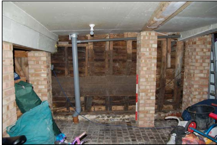
Plate 4: South wall of former stable
