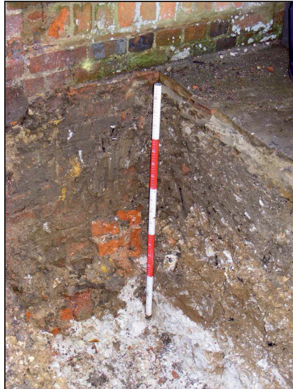
Plate 4: House footings on chalk natural. ( Scale = 1m )
