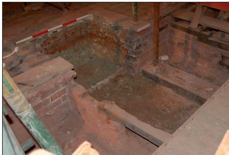
Plate 7: Walls within the internal trench
