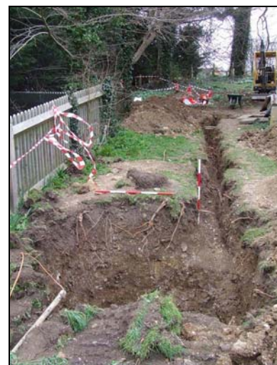
Plate 6: Cess pit and trench, facing North
