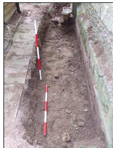
Plate 12: French drain, facing East
