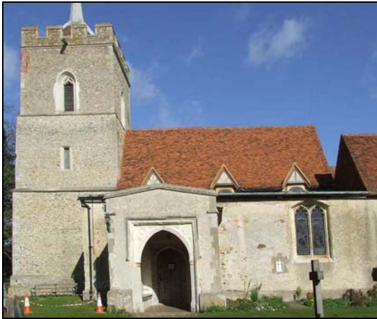
Plate 1: St Mary's Church, Aspenden, facing North
