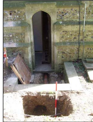
Plate 2: Test pit and drainage run into tower, facing East
