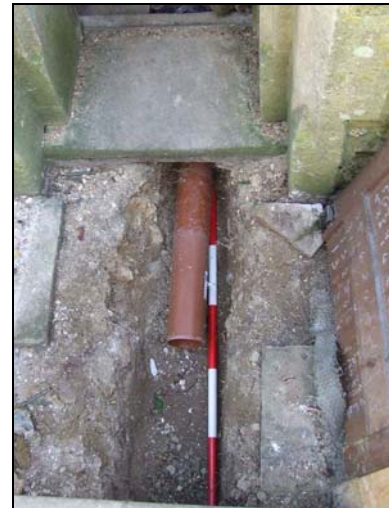
Plate 4: Drainage run under church tower doorway, facing East
