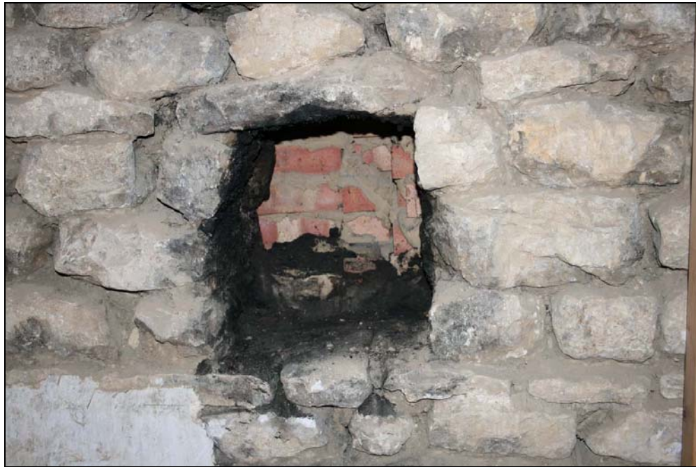
Plate 2: Soot lined cavity in the east wall
