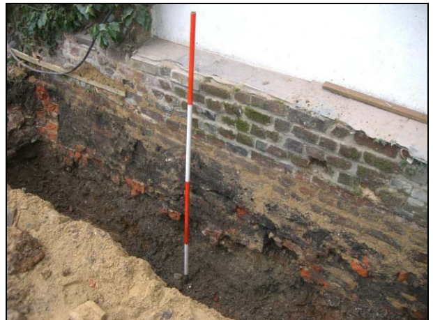
Plate 4: Northernmost foundation adjacent to boundary wall
