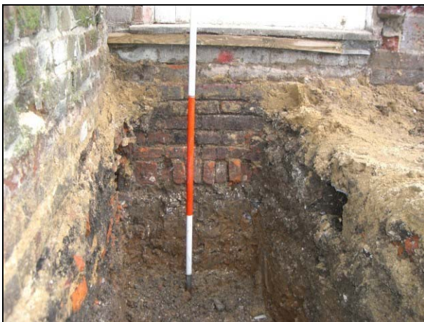
Plate 5: Detail of foundation of existing house on west side
