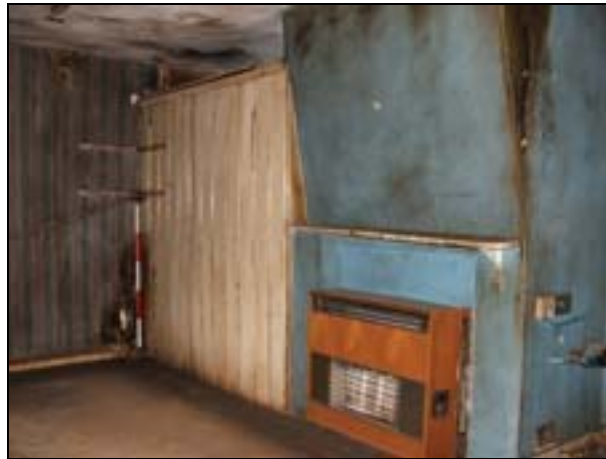
Plate 75: Room S3: northeast corner
