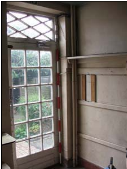
Plate 1: Room G1: SW corner
