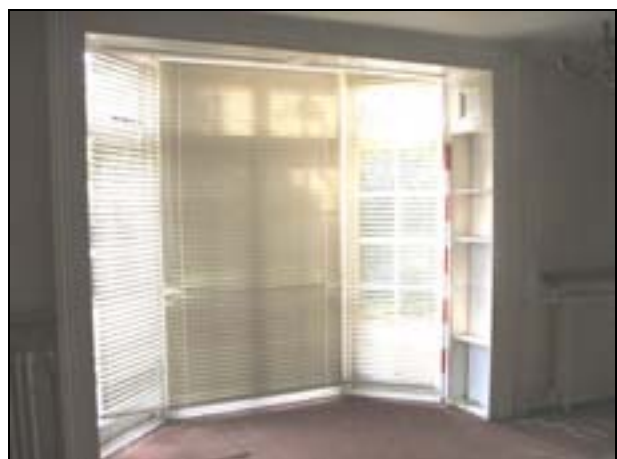
Plate 10: Room G3: south wall
