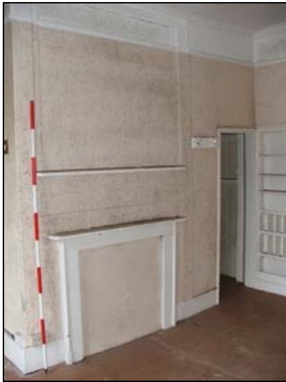
Plate 63: Room F11: north wall
