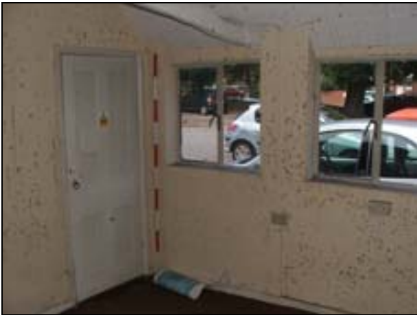
Plate 31: Room G9: northwest corner
