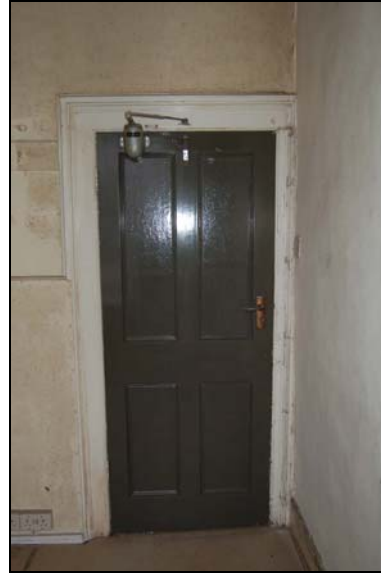
Plate 68: Room F12: south door
