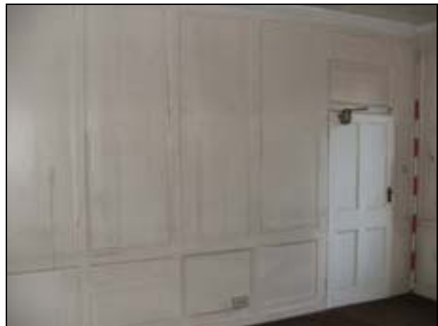
Plate 41: Room G11: south wall
