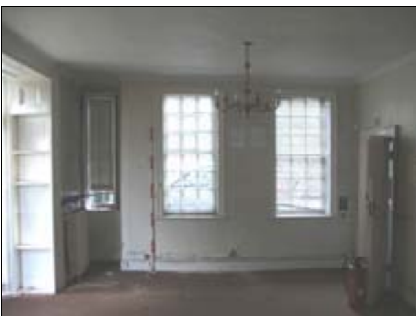
Plate 9: Room G3: west wall
