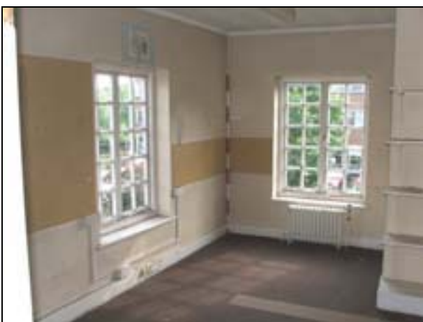
Plate 60: Room F7: SE corner
