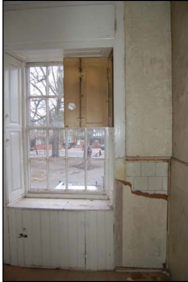
Plate 67: Room F12 showing cupboard, shutters & tiles
