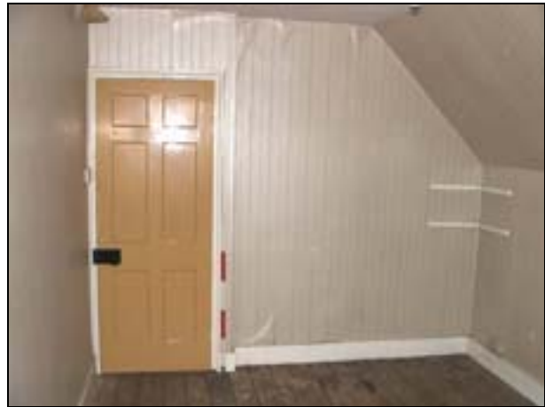
Plate 82: Room S7: west wall
