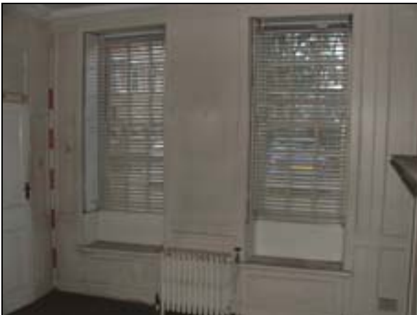
Plate 40: Room G11: west wall
