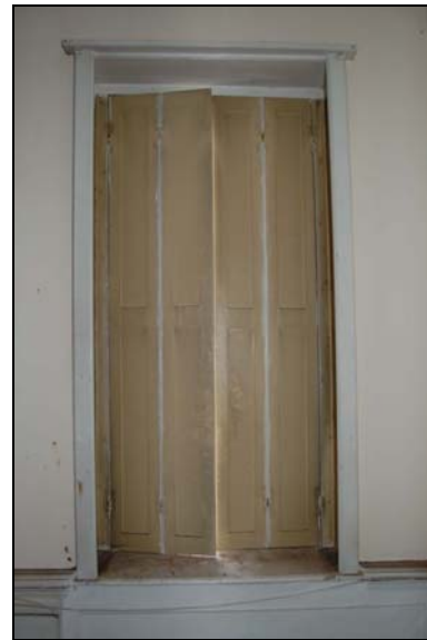
Plate 53: Room F4: replacement shutter
