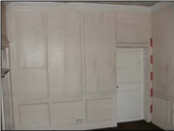
Plate 38: Room G11: east wall
