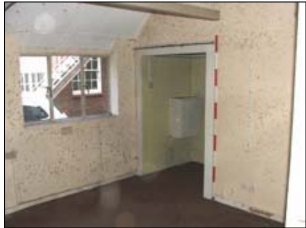
Plate 32: Room G9: northeast corner
