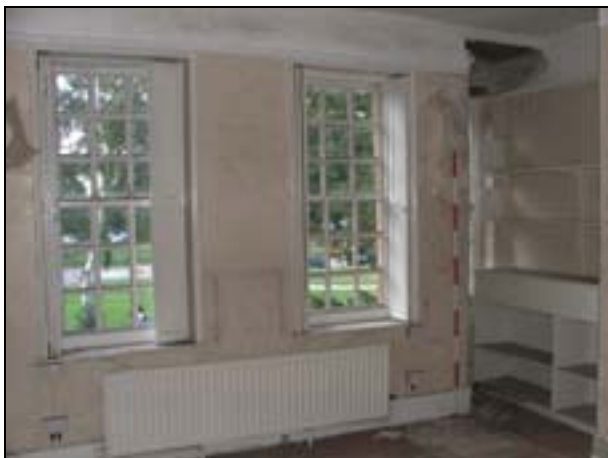
Plate 65: Room F11: west wall
