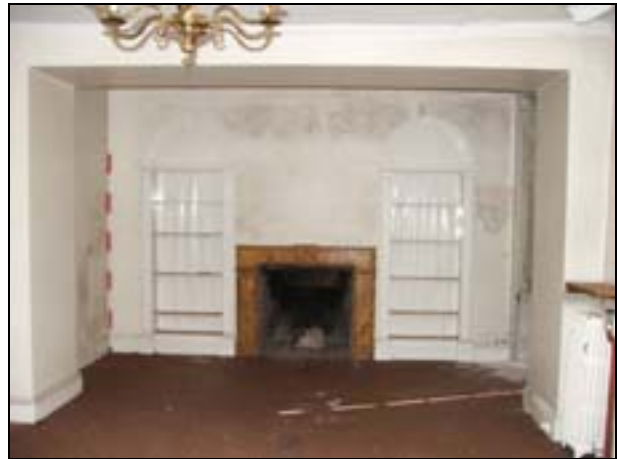
Plate 8: Room G3: east wall
