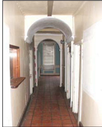
Plate 14: Room G4 showing hatch and 1930s arch
