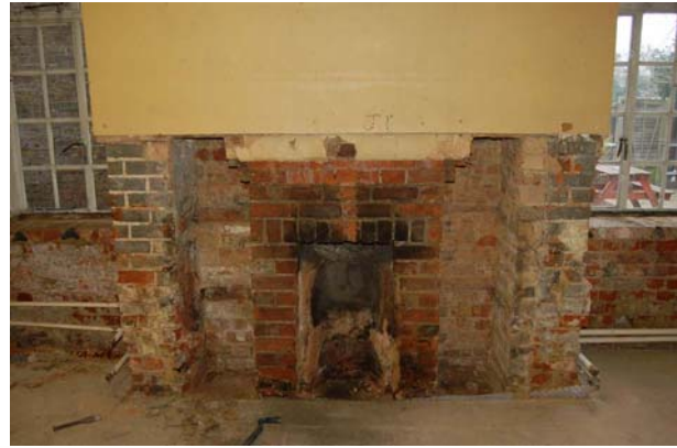
Plate 30: Room G8: fireplace in east wall
