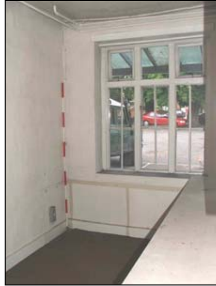
Plate 37: Room G10: north wall
