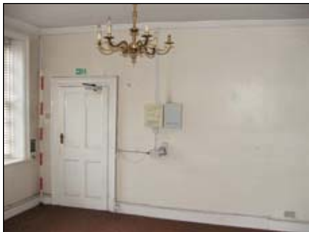
Plate 11: Room G3: north wall
