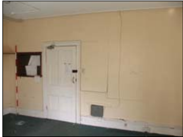
Plate 4: Room G2: north wall
