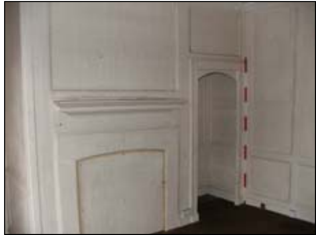
Plate 39: Room G11: north wall
