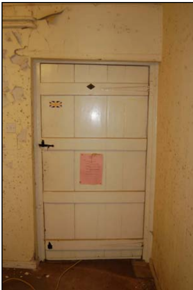
Plate 33: Room G9: interior of door to passage
