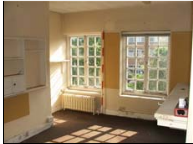
Plate 59: Room F6: south wall
