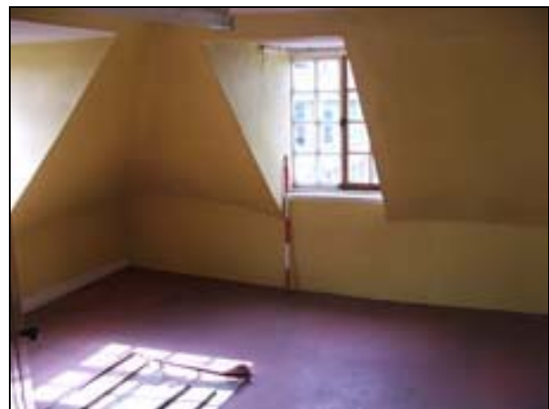
Plate 77: Room S4: west wall
