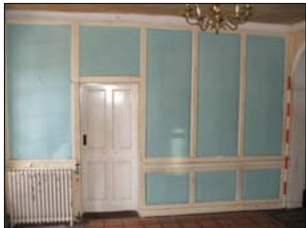
Plate 21: Room G6, north wall
