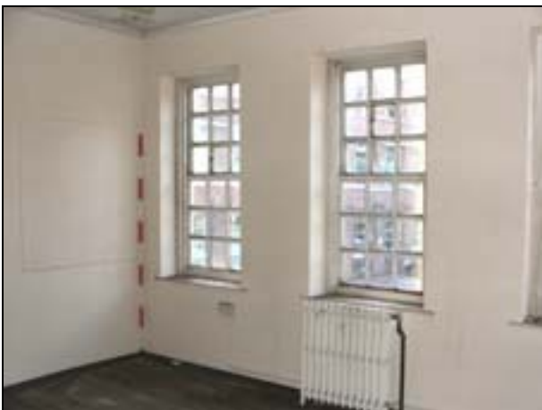
Plate 48: Room F3: SW corner
