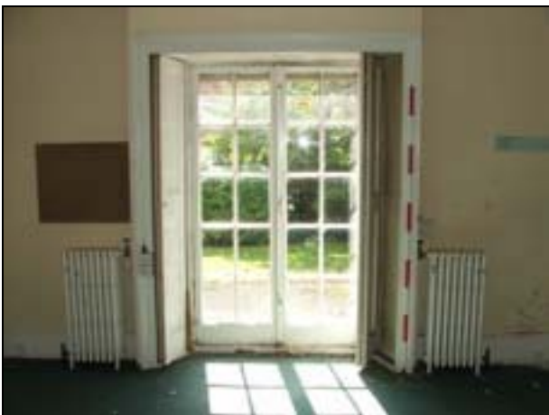
Plate 5: Room G2: south wall
