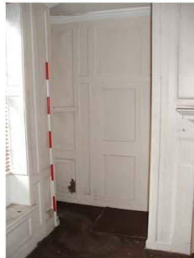
Plate 66: Room F11: northwest corner
