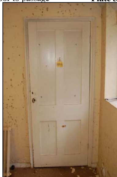
Plate 35: Room G9: door to western cupboard
