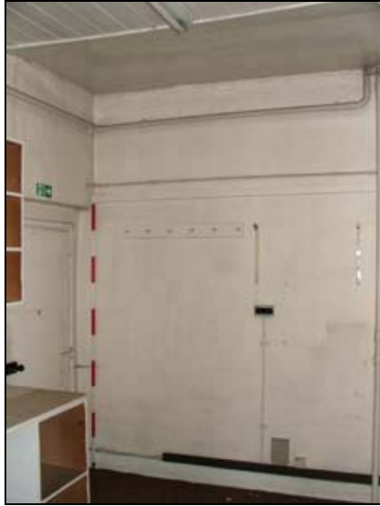
Plate 36: Room G10: south wall
