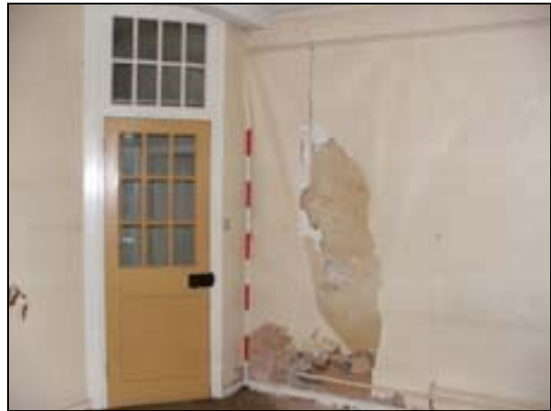
Plate 28: Room G8: northeast corner
