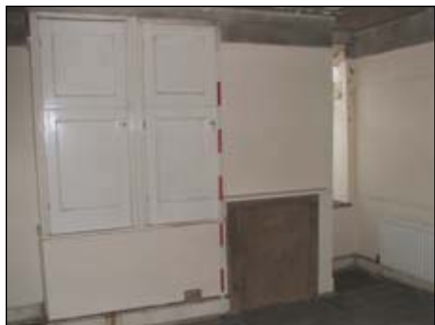
Plate 70: Room F13: east wall
