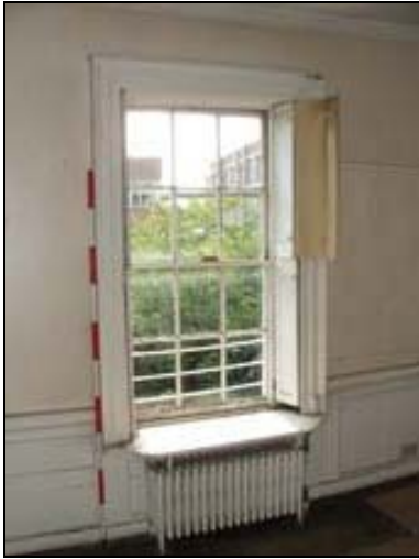
Plate 54: Room F4: south window
