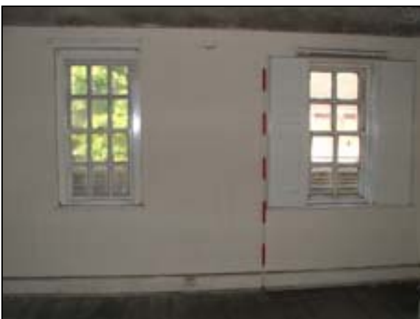
Plate 69: Room F13: north wall
