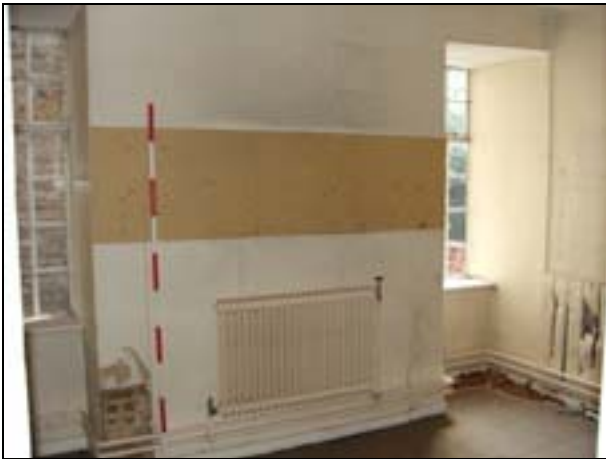
Plate 27: Room G8: SE corner
