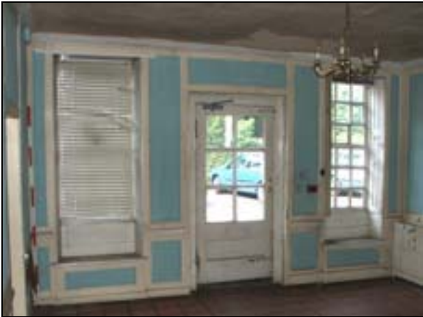
Plate 18: Room G6, west wall
