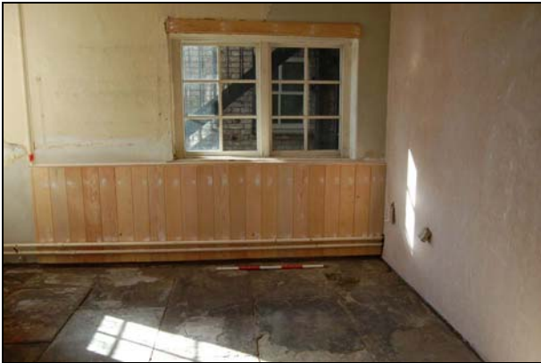
Plate 29: Room G8: west wall undergoing restoration
