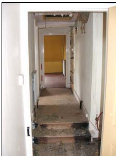
Plate 83: Room S8 looking west
