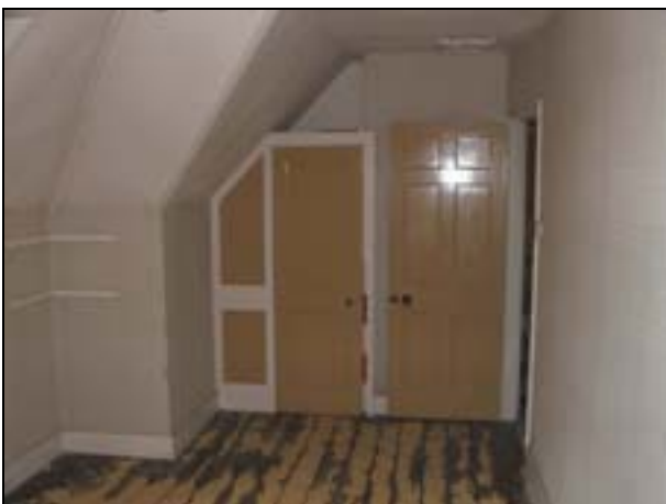
Plate 79: Room S6: west wall & 1930s cupboards
