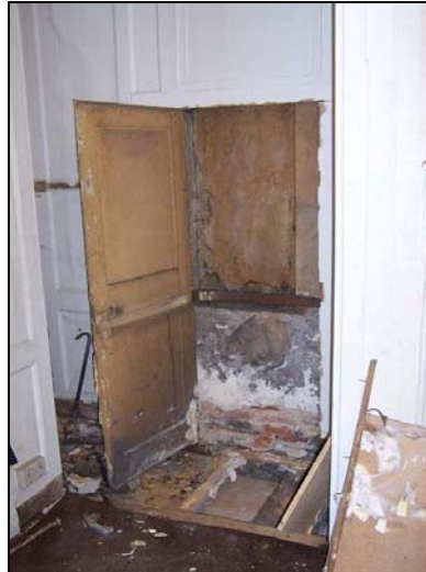
Plate 42: Room G11: northwest recess during restoration
