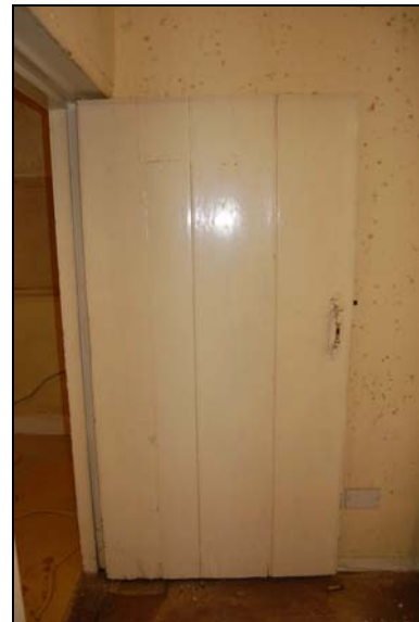
Plate 34: Room G9: door to passage
