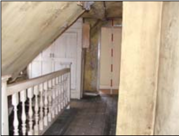
Plate 71: Room S1 looking south
