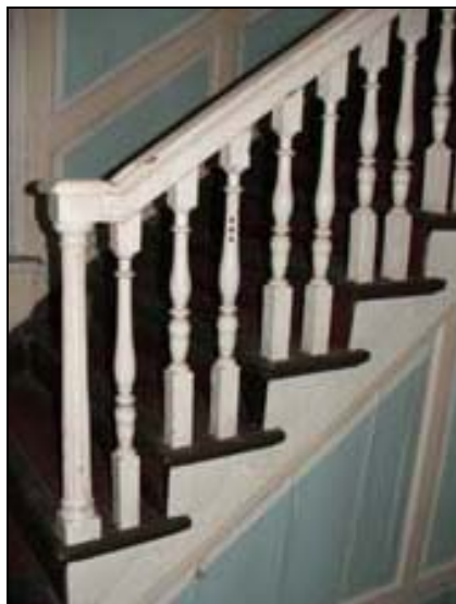
Plate 23: Room G6: stair detail
