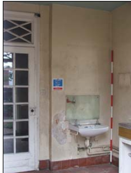
Plate 2: Room G1: NE corner
