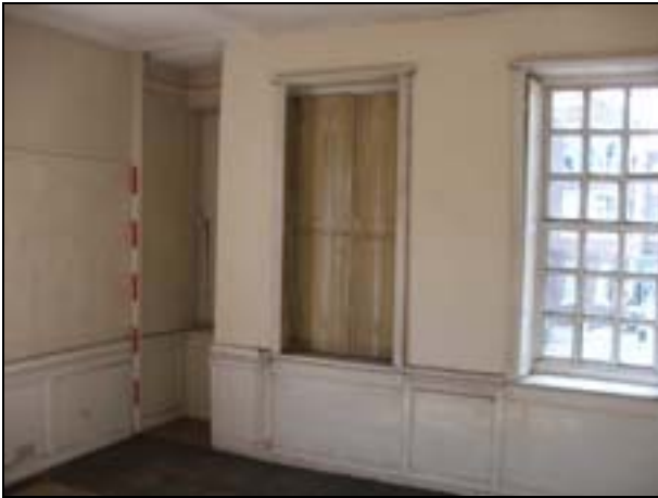
Plate 50: Room F4: SW corner
