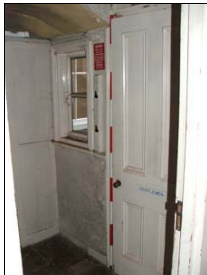
Plate 17: Room G5 looking northeast
