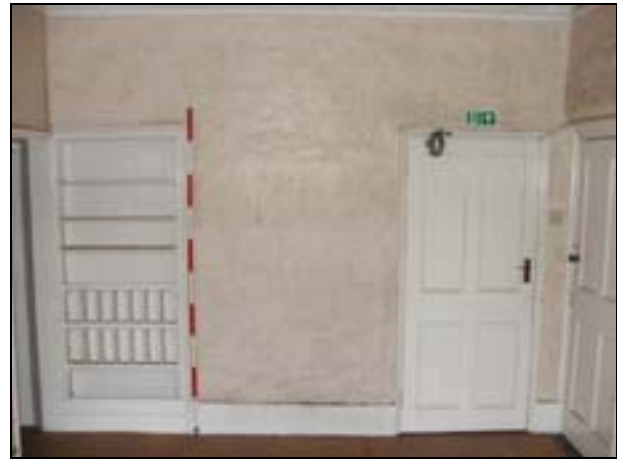
Plate 64: Room F11: east wall showing modern shelving & 1930s door
