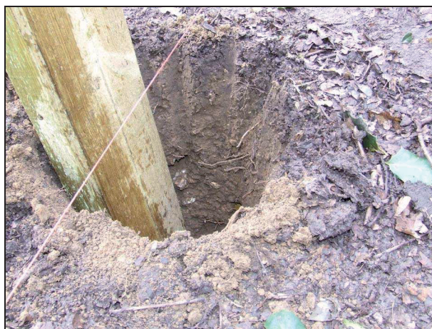
Plate 3: Typical post hole
