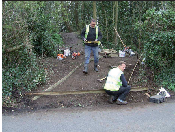
Plate 1: Construction of the ramp access
