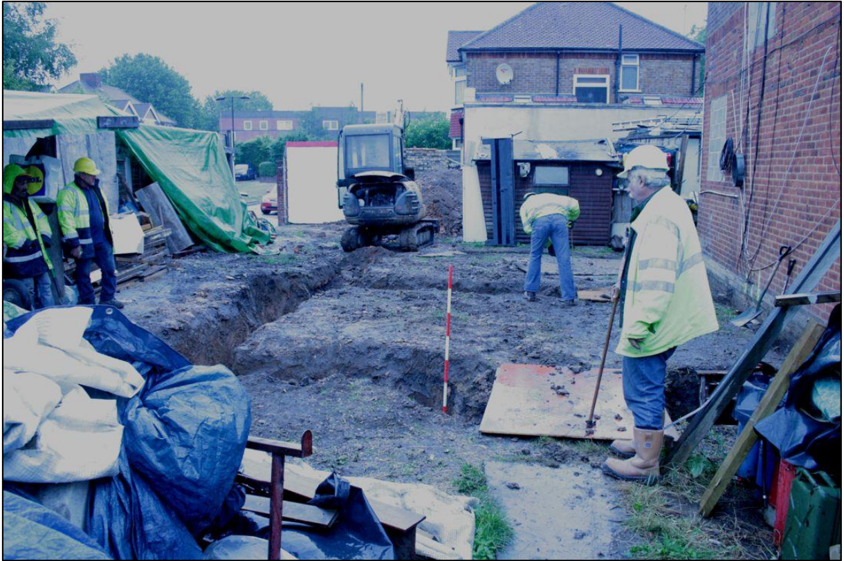
Plate 1: General view of site, looking north
