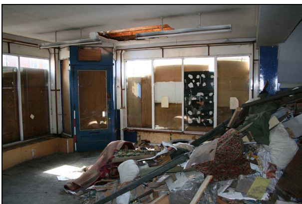
Plate 11: Room G1: northeast corner
