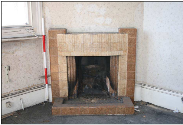
Plate 31: Room F1: fireplace detail
