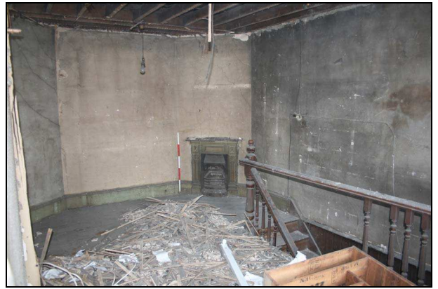
Plate 32: Room F2: southwest corner
