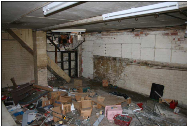
Plate 9: Cellar: northwest corner
