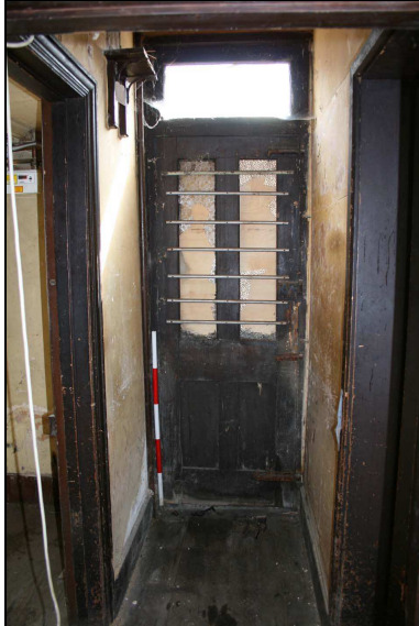
Plate 21: Room G3: east wall
