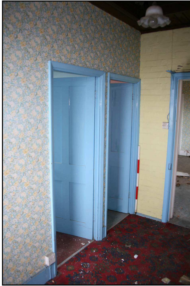
Plate 43: Room F6: northwest corner
