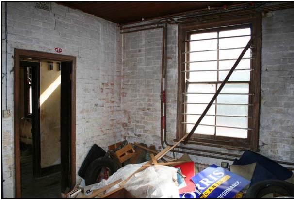
Plate 25: Room G4: northeast corner
