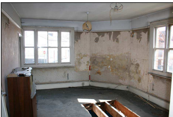
Plate 29: Room F1: north wall
