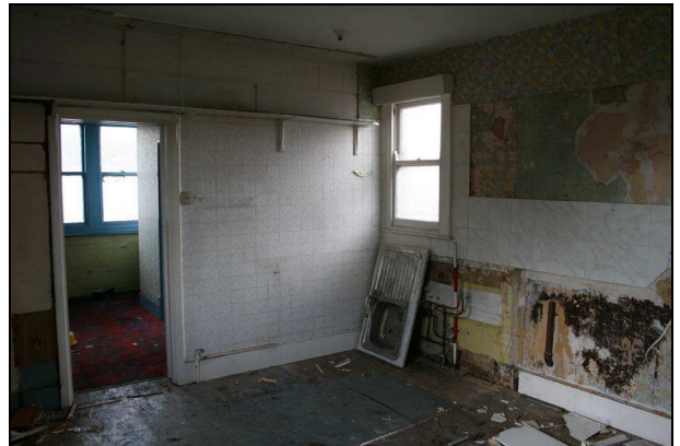
Plate 40: Room F5: southwest corner
