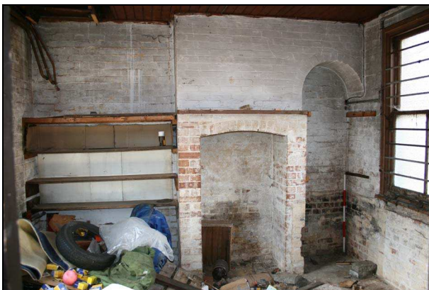
Plate 23: Room G4: south wall
