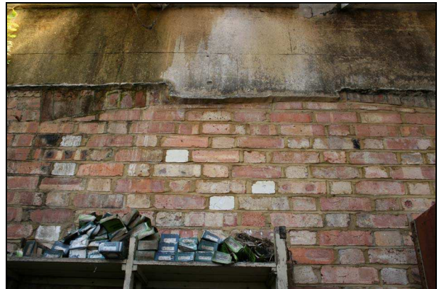
Plate 28: Room G6: north wall detail showing relieving arch, later brickwork & render
