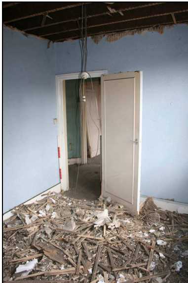
Plate 39: Room F4: northwest corner
