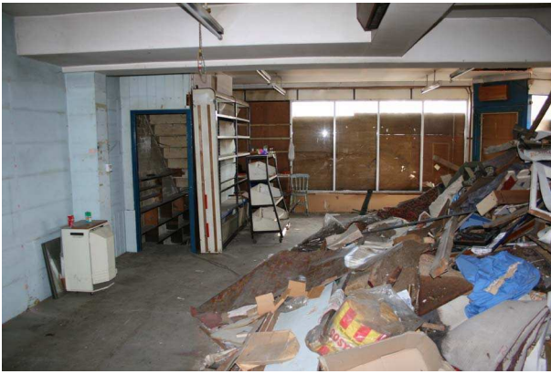
Plate 13: Room G1: west wall
