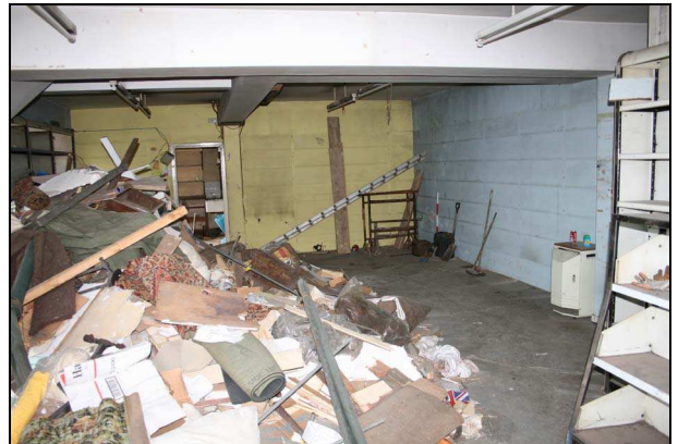
Plate 10: Room G1: looking south
