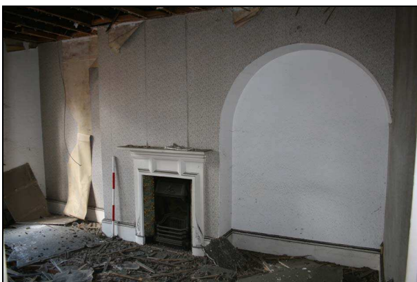
Plate 35: Room F3: northwest corner
