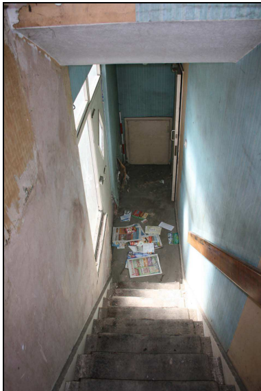
Plate 27: Room G5: looking south
