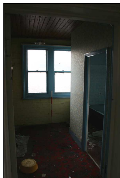
Plate 42: Room F6: looking south
