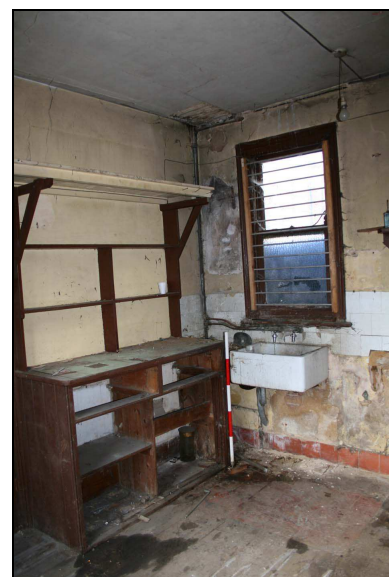
Plate 18: Room G2: southwest corner
