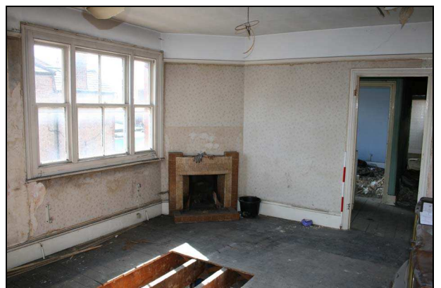
Plate 30: Room F1: southeast corner
