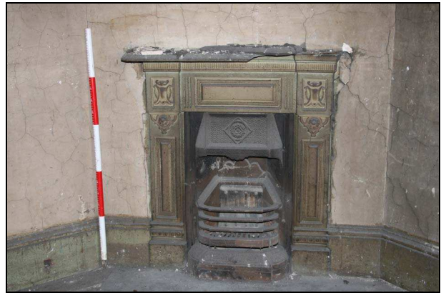
Plate 34: Room F2: fireplace detail
