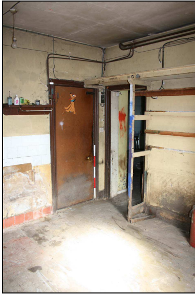
Plate 19: Room G2: northwest corner
