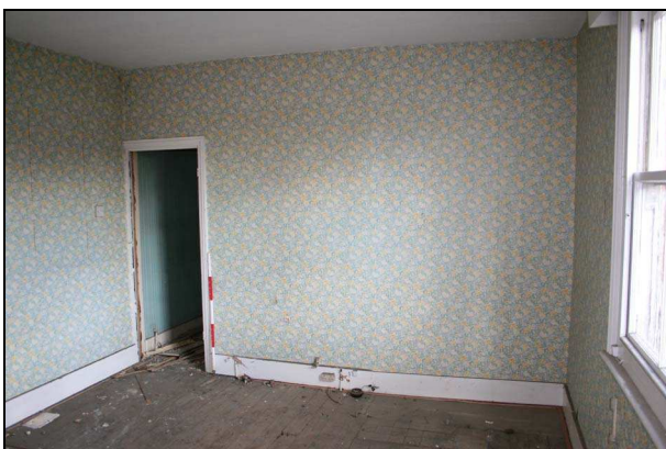
Plate 41: Room F5: north wall
