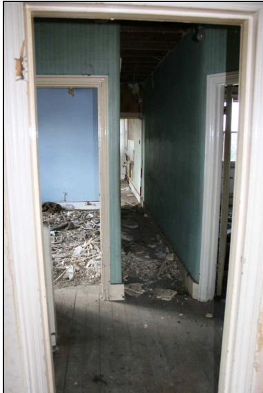
Plate 45: Room F7: looking south
