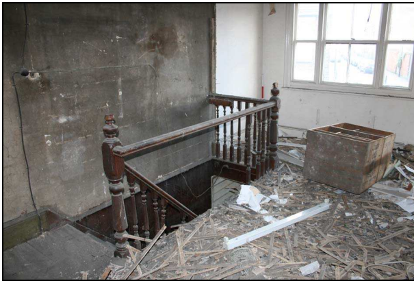
Plate 33: Room F2: northwest corner
