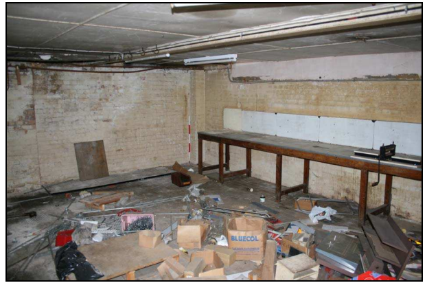
Plate 8: Cellar: southeast corner
