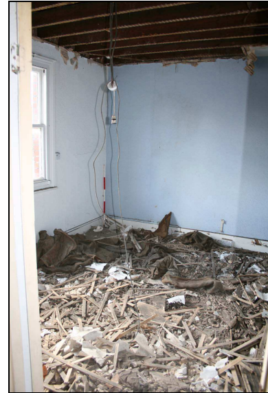
Plate 38: Room F4: southeast corner
