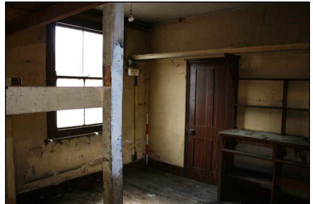
Plate 16: Room G2: southeast corner
