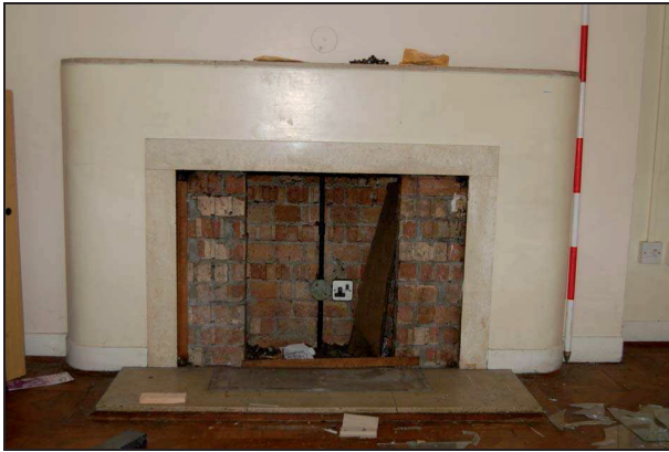
Plate 175: Room G3: fireplace detail
