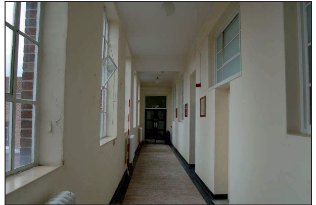
Plate 141: Corridor S8: looking east
