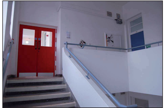
Plate 129: Stairwell S2: north wall
