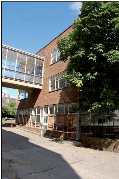
Plate 222: North Range: west elevation
