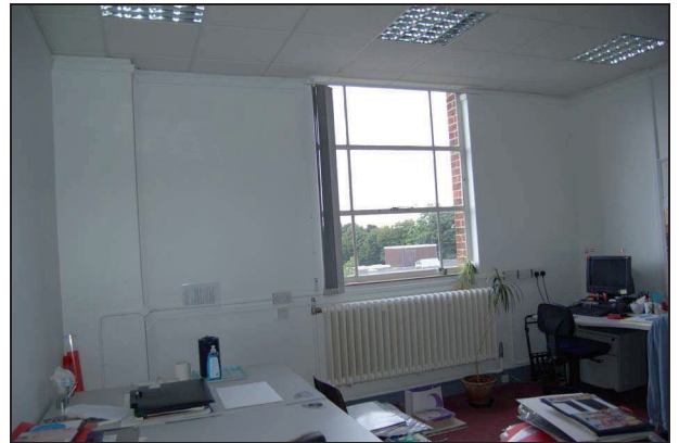
Plate 131: Room S3: east wall
