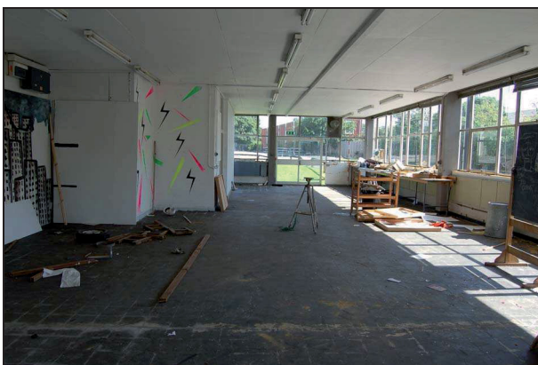
Plate 236: Room G4: north wall
