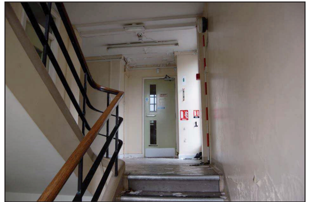
Plate 208: Stairwell F6: east wall
