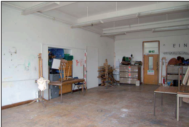
Plate 88: Room F2: southeast corner
