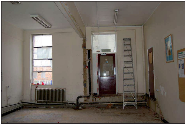
Plate 94: Room F6: east wall
