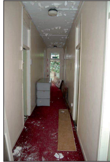
Plate 194: Corridor G11 southern end: looking south
