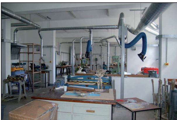
Plate 60: Room G18: looking north
