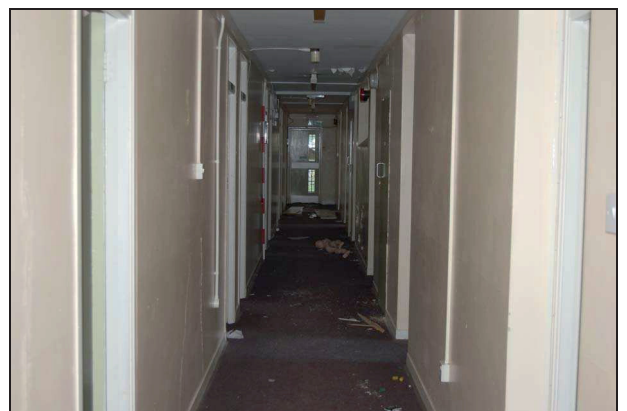
Plate 198: Corridor F1: looking west
