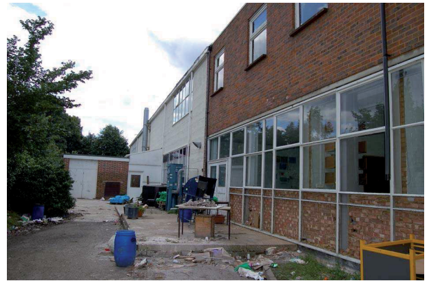
Plate 229: East Range: east elevation (looking south)
