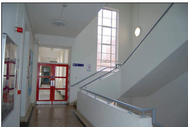
Plate 84: Eastern stairwell (F1): looking east
