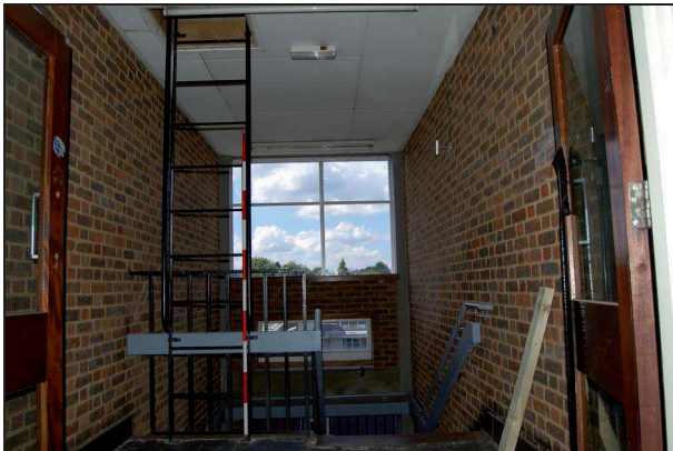
Plate 246: Stairwell (S2): looking south
