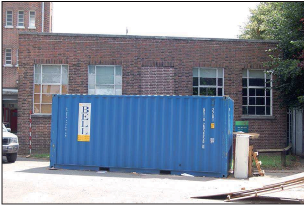
Plate 20: Maintenance Block: west elevation
