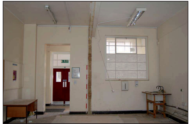
Plate 95: Room F6: west wall
