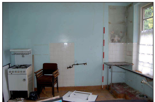
Plate 186: Room G9: west wall
