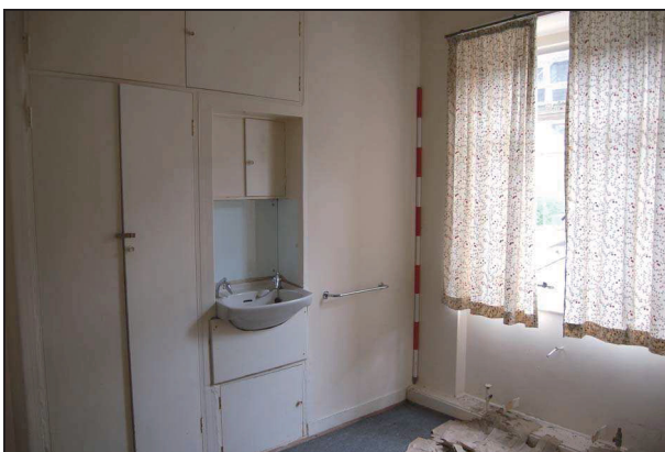
Plate 197: Room G14: southwest corner
