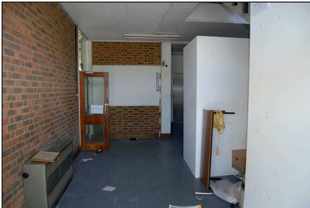
Plate 240: Main entrance (G7): north wall
