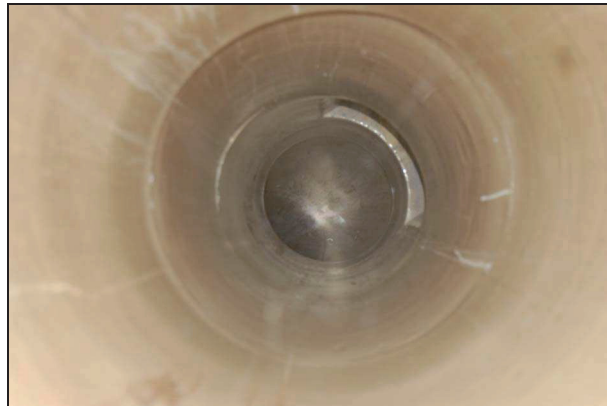
Plate 219: Stairwell S3: view down the chute
