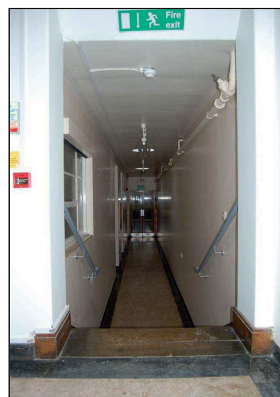
Plate 121: Corridor F21: looking north
