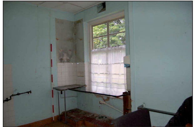
Plate 188: Room G9: northwest corner
