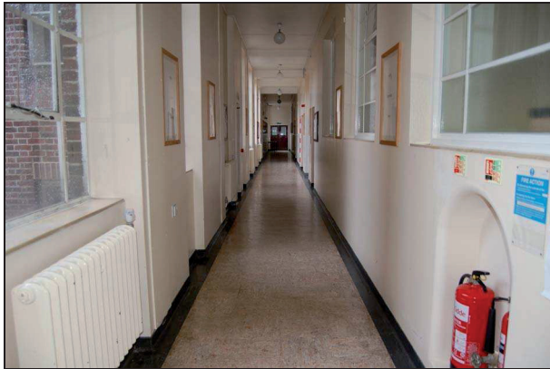
Plate 116: Corridor F18: looking south
