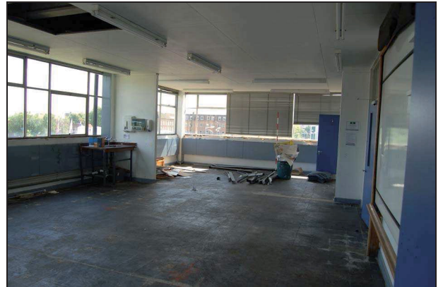
Plate 245: Room S1: looking east
