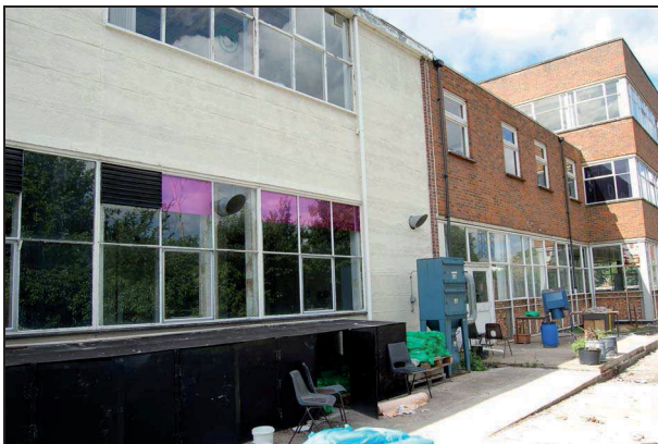
Plate 228: East Range: east elevation (looking northwest)
