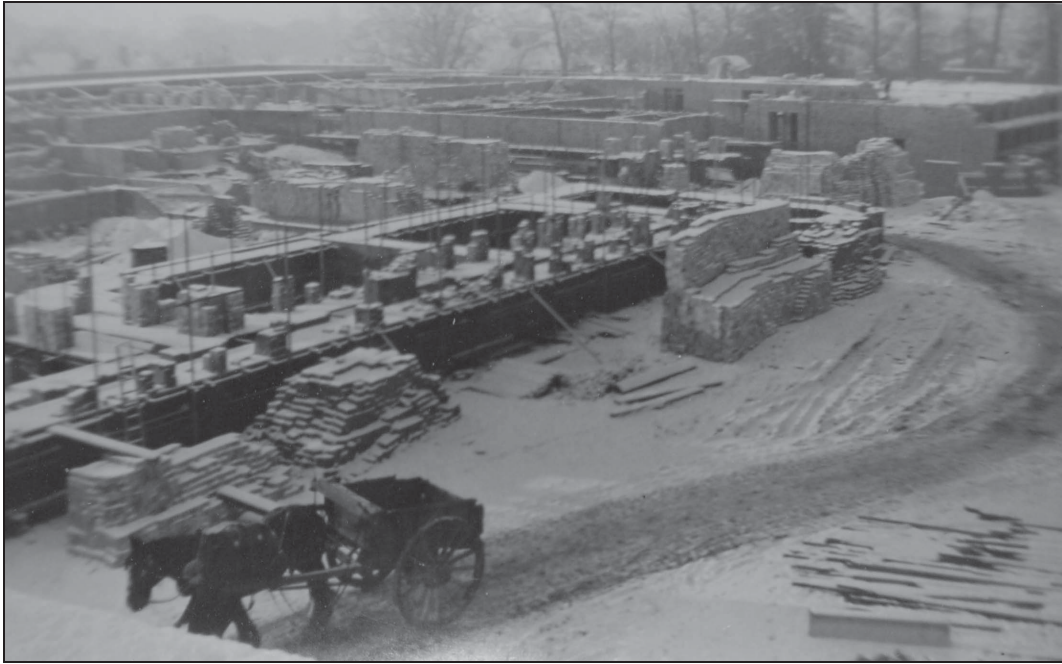
Plate 2: Building works, December 29 th 1939
