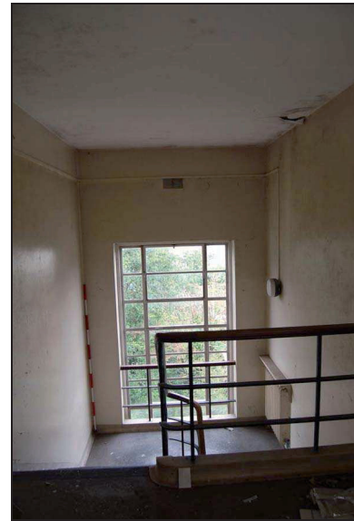
Plate 218: Stairwell S3: east wall
