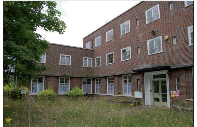
Plate 158: North elevation: looking southeast
