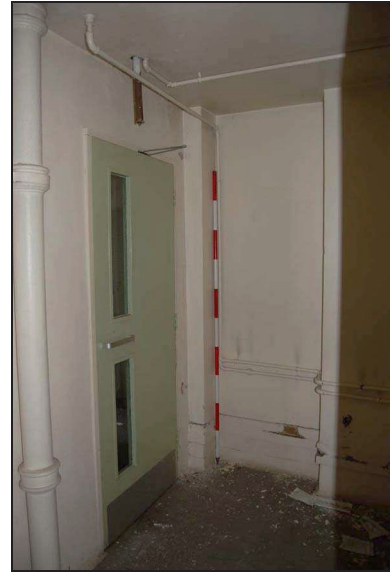
Plate 206: Room F5: looking northwest
