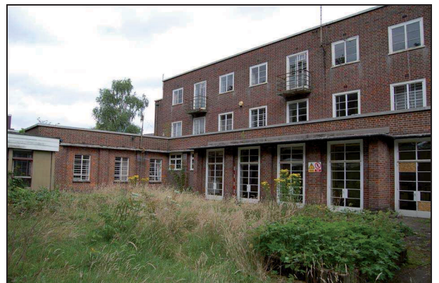
Plate 162: South elevation: looking northwest
