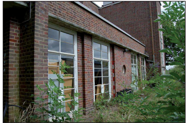
Plate 166: East elevation: southern end
