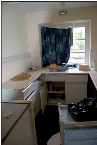
Plate 213: Room F9: west wall
