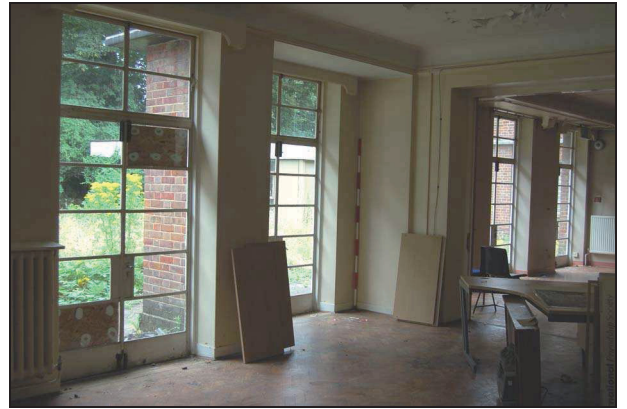
Plate 176: Room G3: looking southwest
