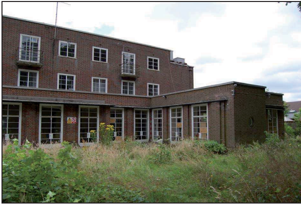
Plate 163: South elevation: looking northwest
