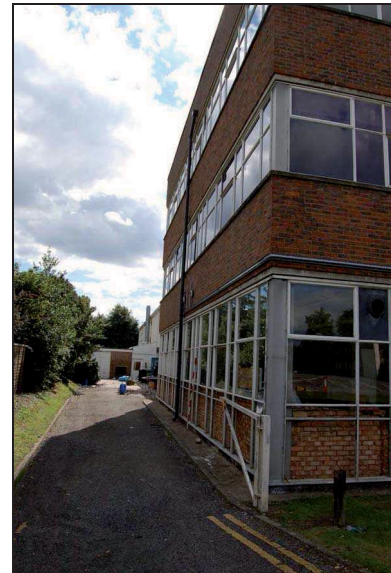
Plate 223: North Range: east elevation
