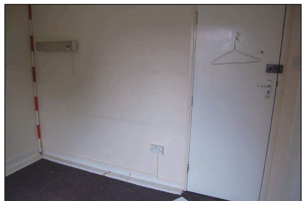
Plate 210: Room F7: southeast corner
