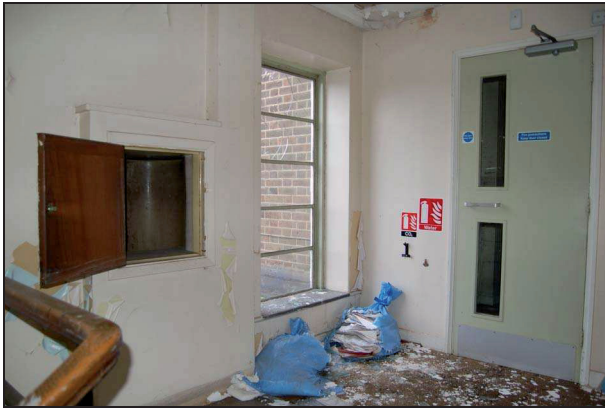
Plate 217: Stairwell S3: southwest corner
