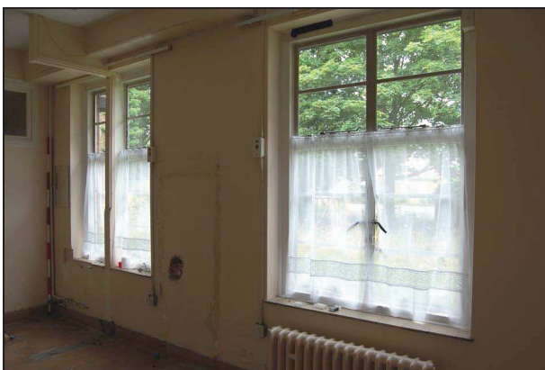
Plate 185: Room G8: looking northwest
