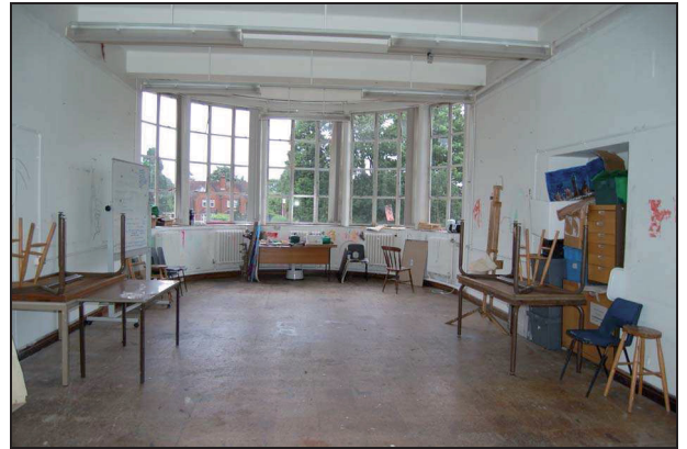
Plate 87: Room F2: north wall
