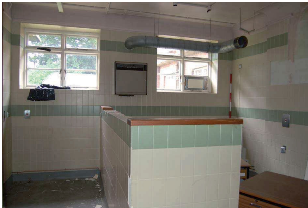
Plate 177: Room G5: southwest corner
