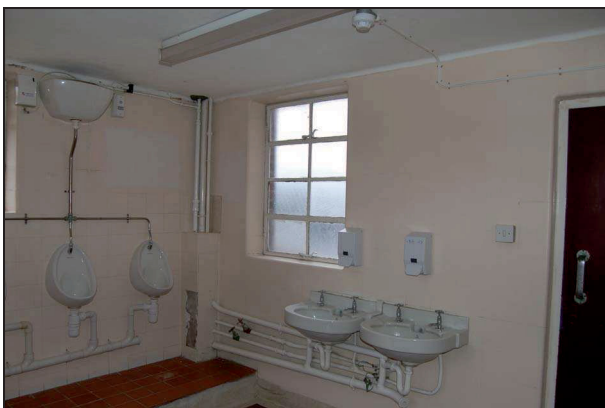
Plate 102: Room F10: southwest corner
