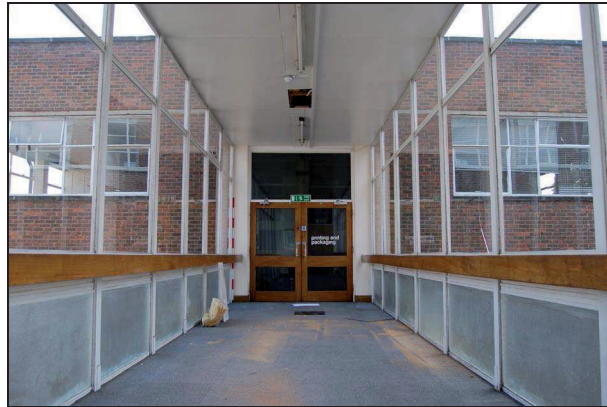
Plate 250: Bridge Passage (S4): looking east
