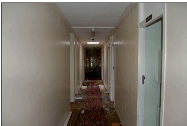
Plate 215: Corridor S1: looking west
