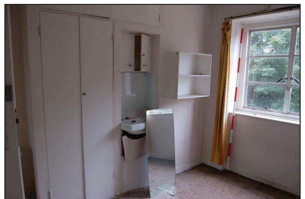
Plate 216: Room S2: southeast corner
