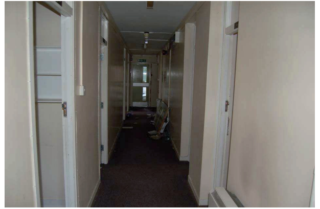
Plate 212: Corridor F8: looking south
