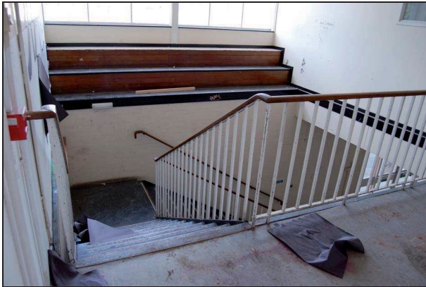
Plate 244: Stairwell F3: looking southwest
