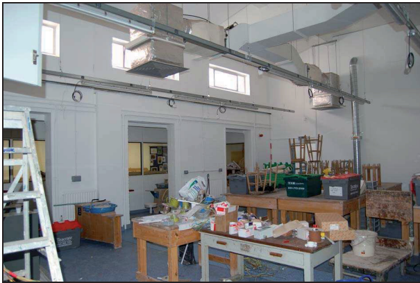
Plate 52: Room G14: northwest corner
