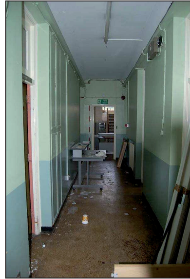
Plate 182: Corridor G7: looking west
