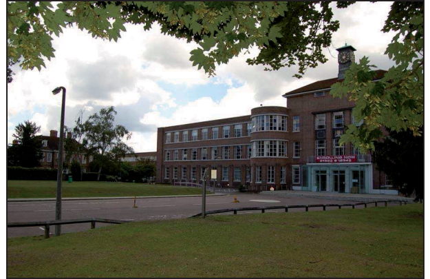
Plate 15: North elevation looking southeast
