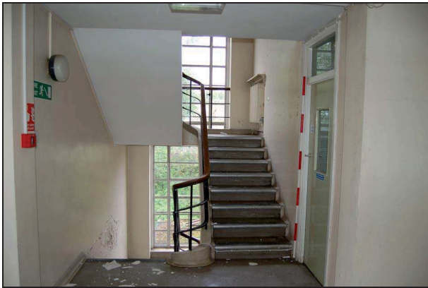
Plate 207: Stairwell F6: west wall
