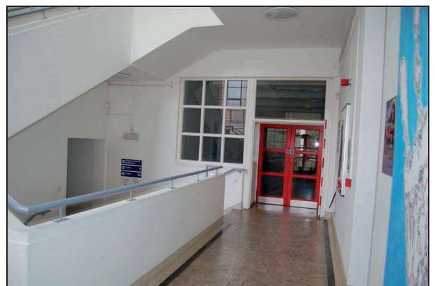
Plate 85: Eastern stairwell (F1): looking west
