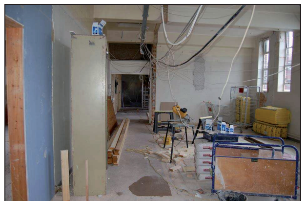
Plate 151: Room F14: under construction
