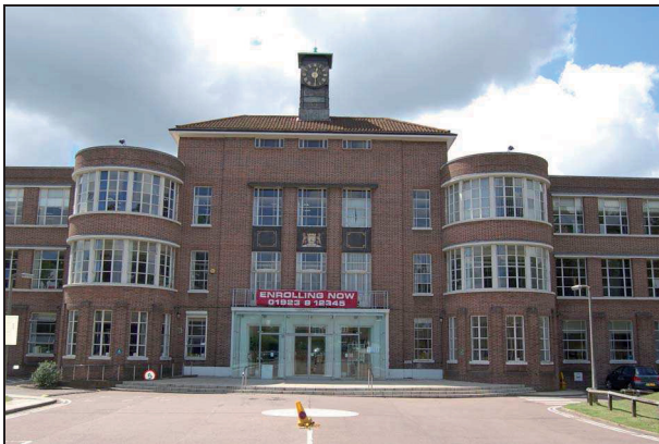
Plate 16: North elevation: central block
