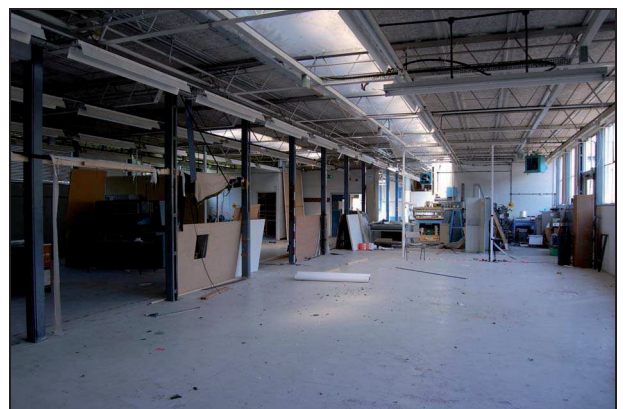
Plate 231: Room G1: looking west
