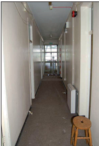
Plate 191: Corridor G11 northern end: looking north
