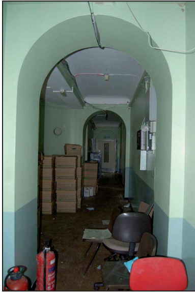
Plate 181: Corridor G7: looking east
