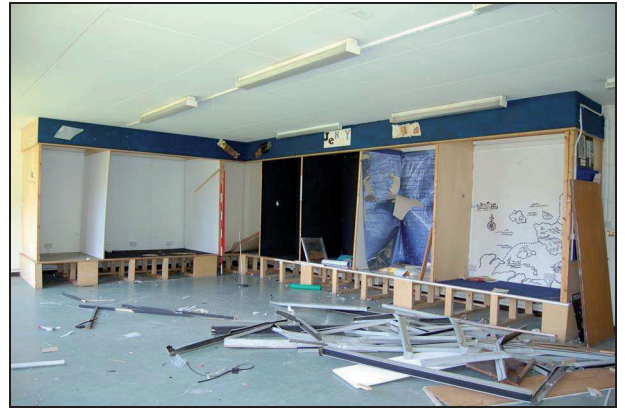
Plate 239: Room G6: looking southeast
