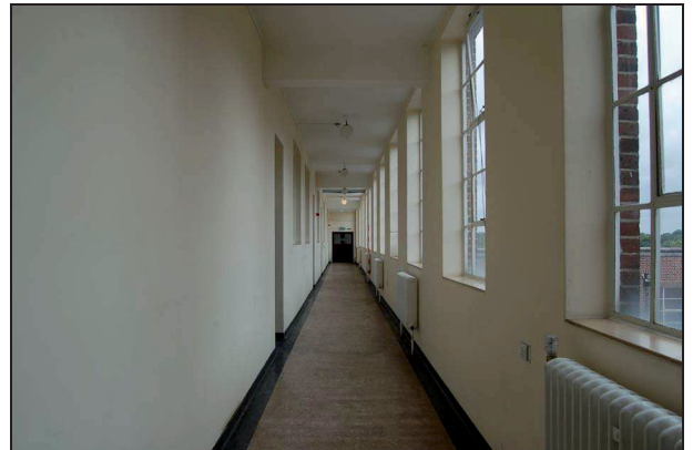
Plate 137: Corridor S5: looking south
