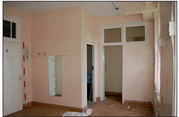
Plate 184: Room G8: west wall
