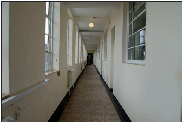
Plate 136: Corridor S5: looking north
