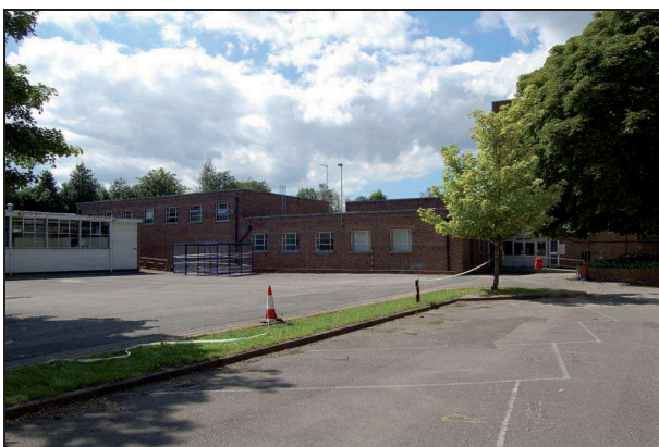
Plate 24: East elevation: southern end
