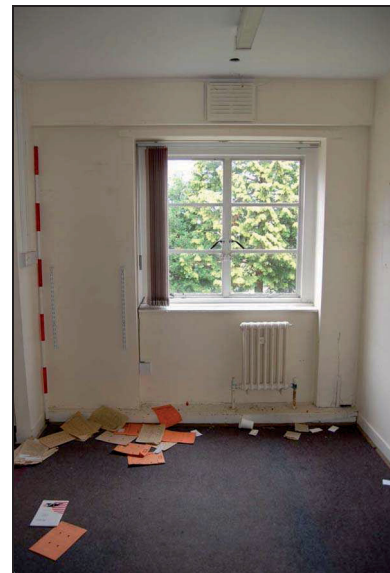
Plate 202: Room F3: north wall
