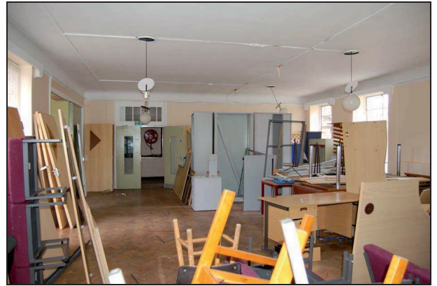
Plate 170: Room G1: north wall
