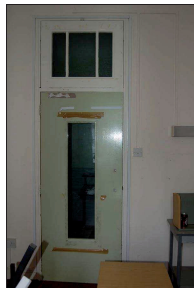
Plate 180: Room G6: south wall
