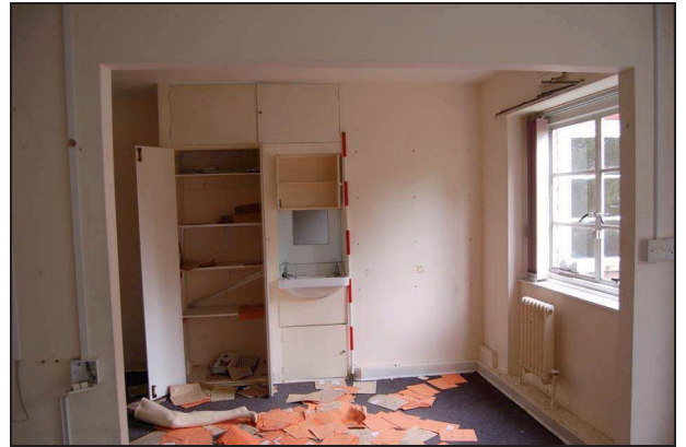
Plate 200: Room F2: west wall
