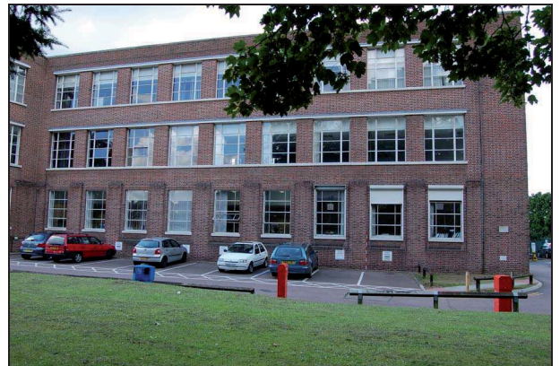
Plate 17: North elevation: western end
