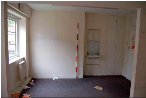
Plate 201: Room F3: east wall
