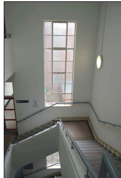
Plate 143: Stairwell S9: half landing to east
