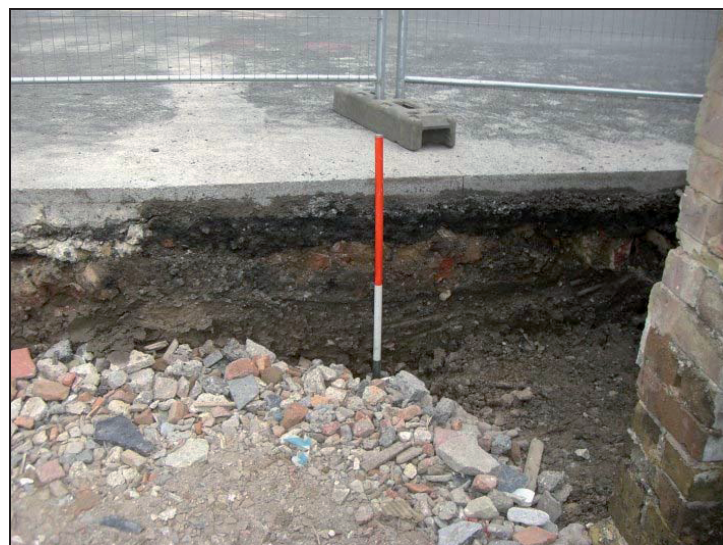
Plate 4: View east of layers beneath the existing ground surface.
