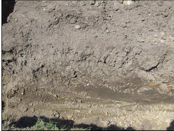
Plate 1: South facing section of southern footing trench
