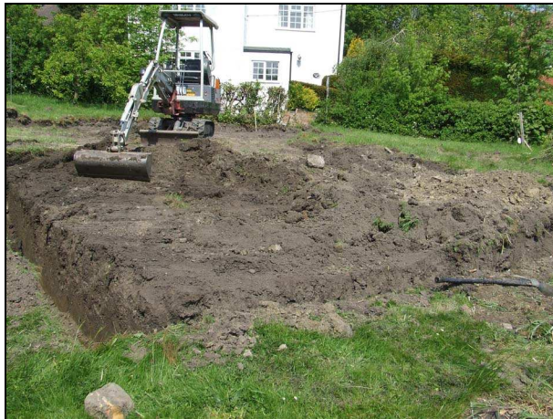
Plate 2: Footing trenches and footprint of new garage
