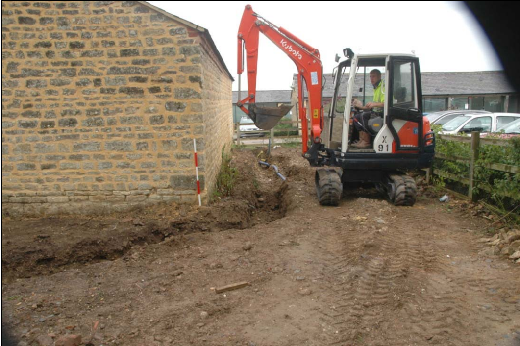
Plate 11: Trench to the east of the easternmost barn
