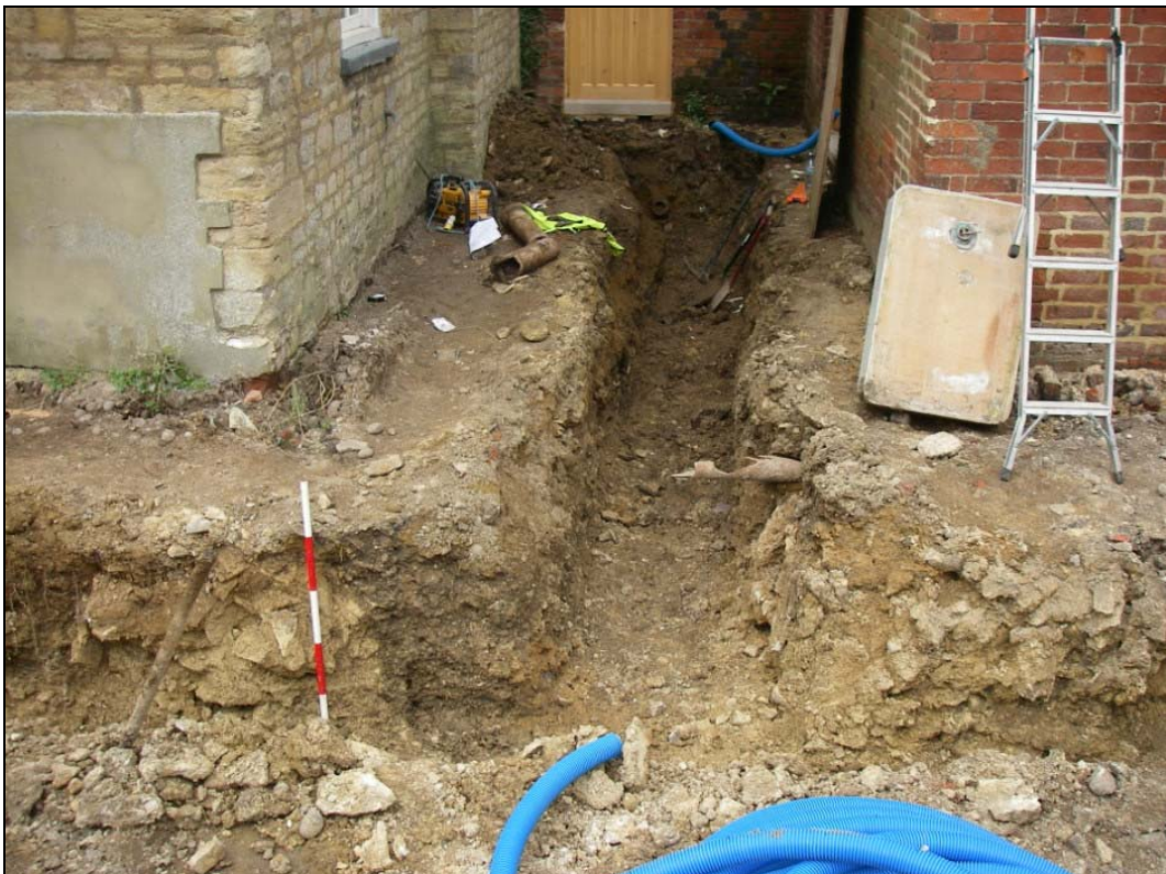
Plate 10: Old service trench on the west side of the courtyard
