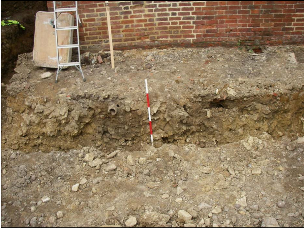
Plate 9: Old service pipe and trench in the courtyard
