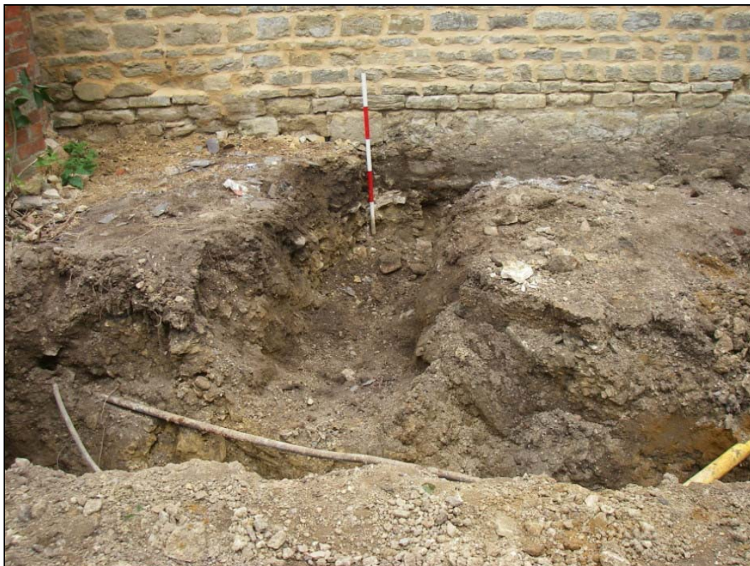
Plate 6: Eastern barn south facing wall footings
