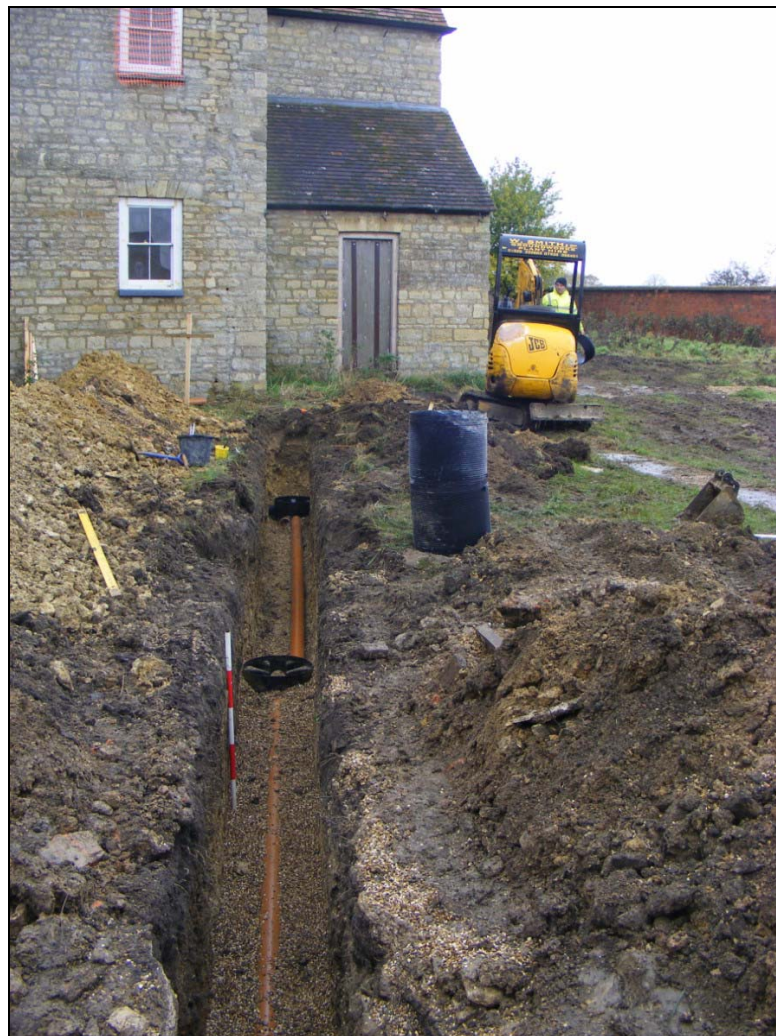
Plate 12: Trench running from the NW corner of the house
