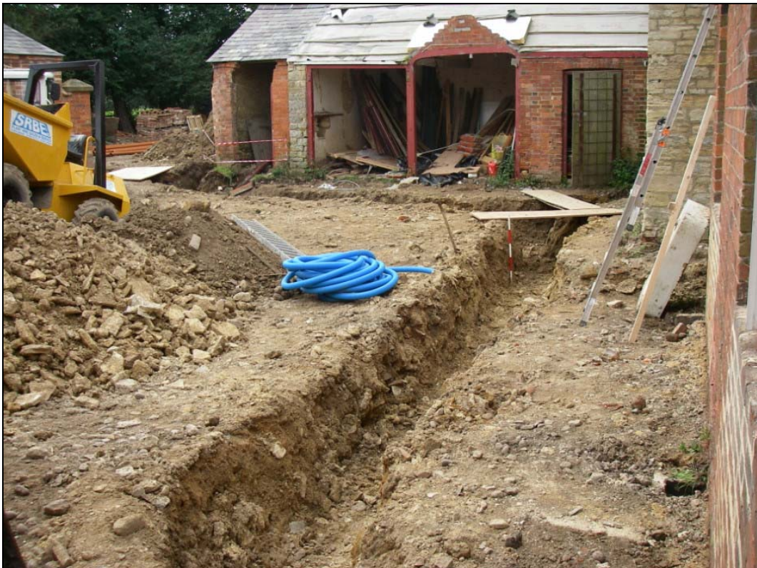
Plate 8: Trench in the main courtyard
