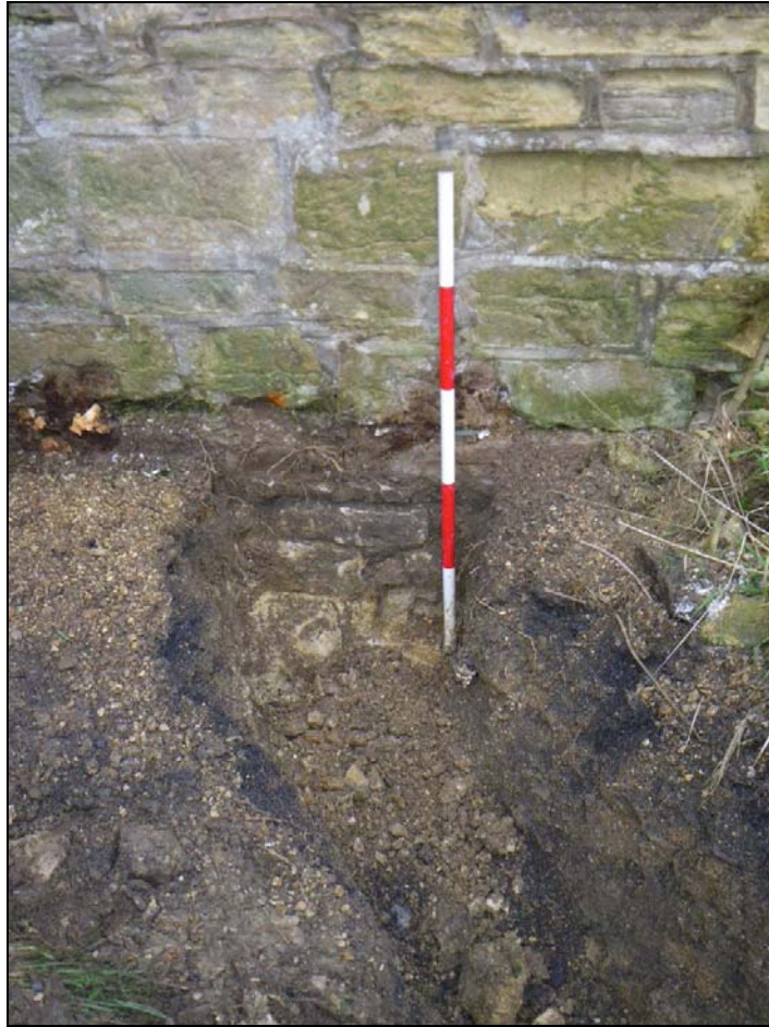
Plate 5: House footings (NW corner)
