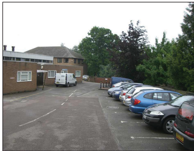
Plate 4: Looking south to Buildings P and T
