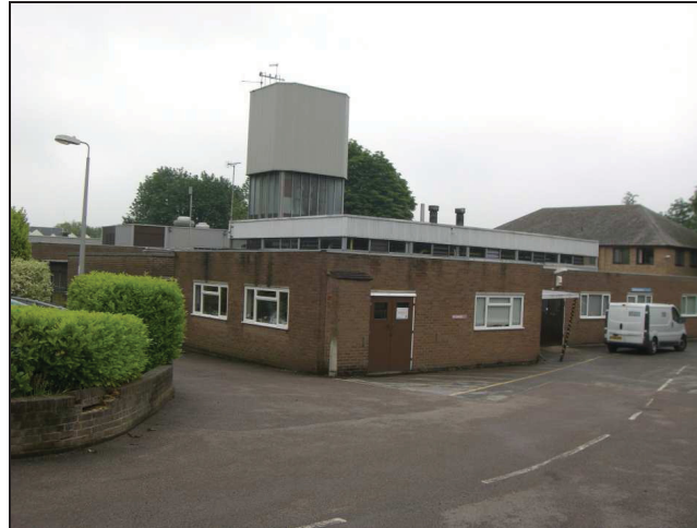
Plate 3: Building P looking southeast
