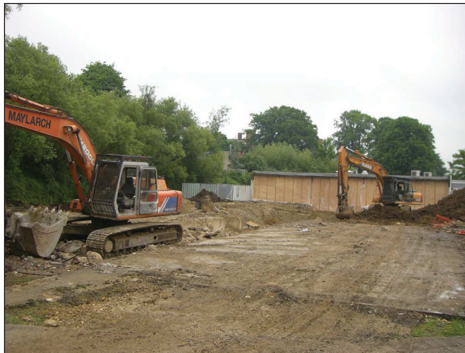
Plate 12: Clearance operations on the site of Building H
