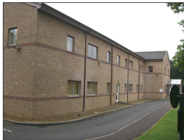
Plate 8: North frontage of Building U looking west
