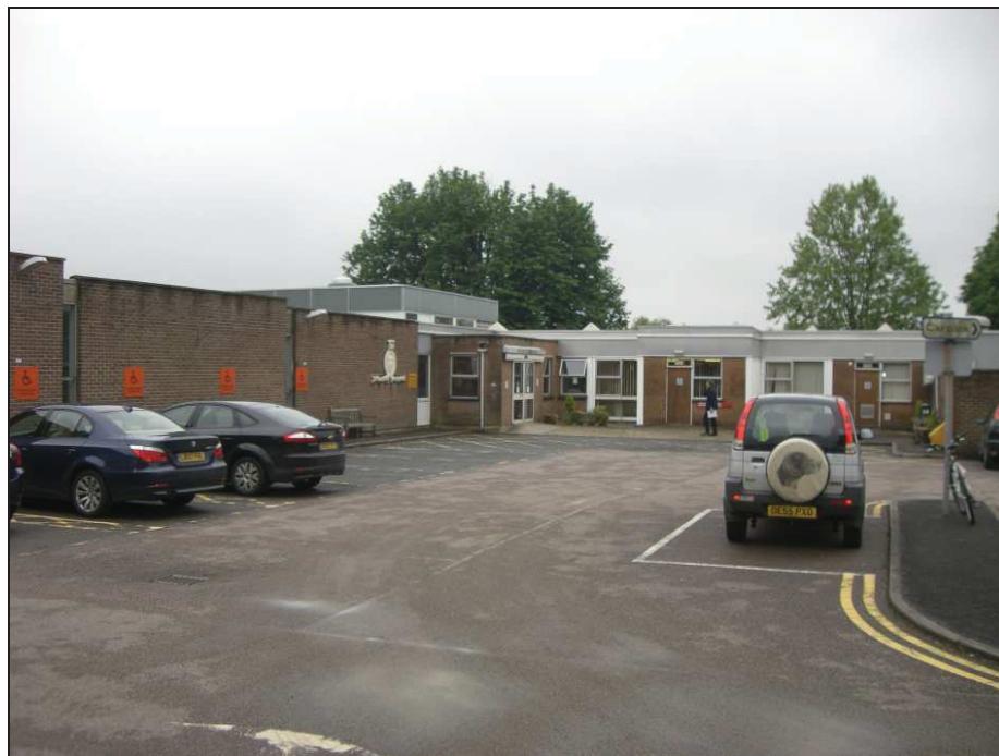
Plate 10: Building L looking south
