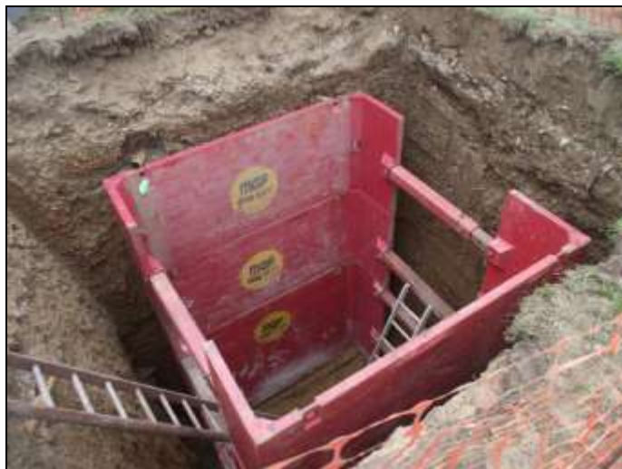
Plate 6: Extension B: northern soakaway
