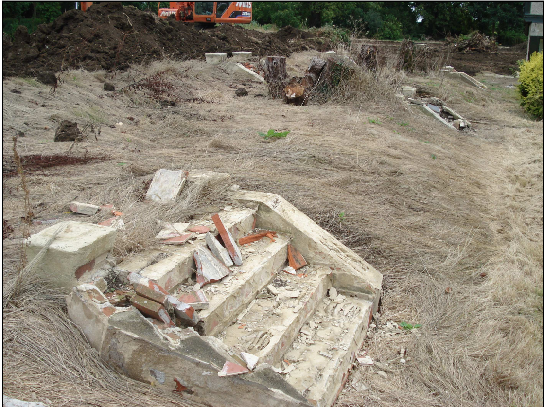
Fig. 2: View from SW end of terrace.
