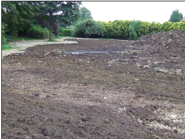
Plate 2: Stripped area showing footpath
