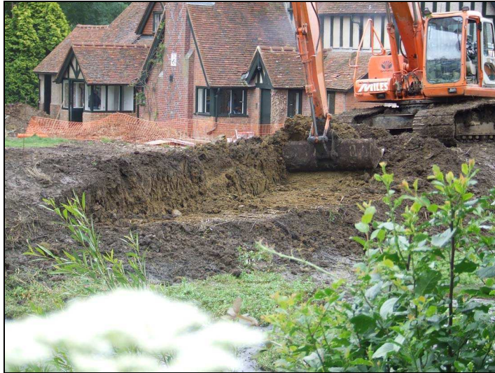
Plate 4: East facing section of pond embankment during groundwork
