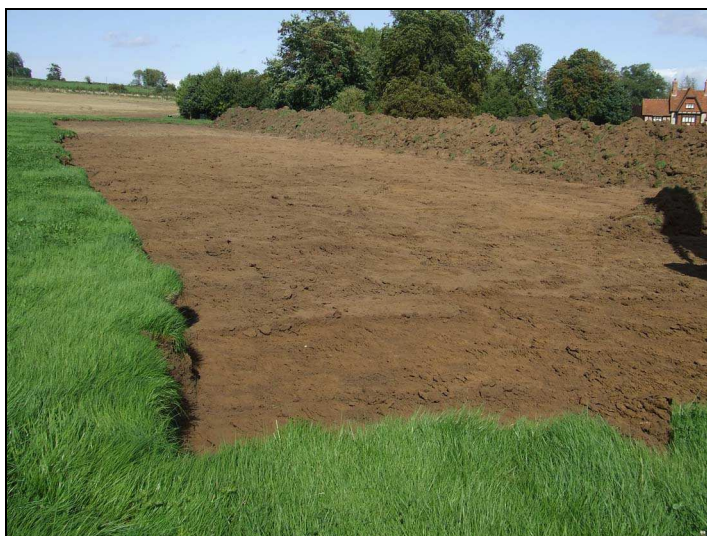
Plate 6: Stripped area of paddock
