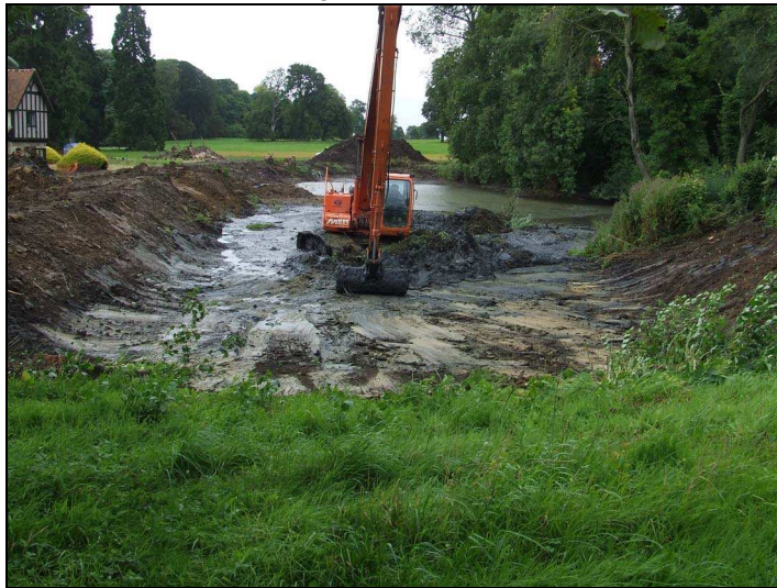
Plate 5: Cleaning northern end of pond
