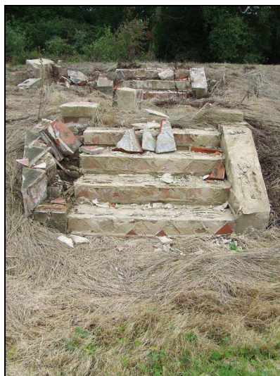
Plate 3: Detail of steps to terrace
