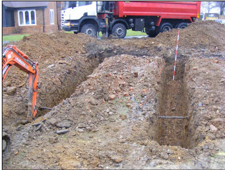
Plate 1: General shot northern square footing trench, looking northeast
